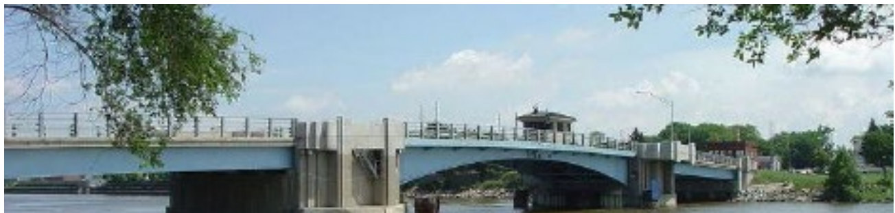
Image Source: Michigan Department of Transportation.
