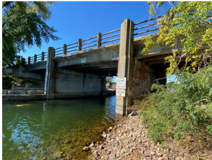
Photo Source: City of Excelsior, Minnesota
