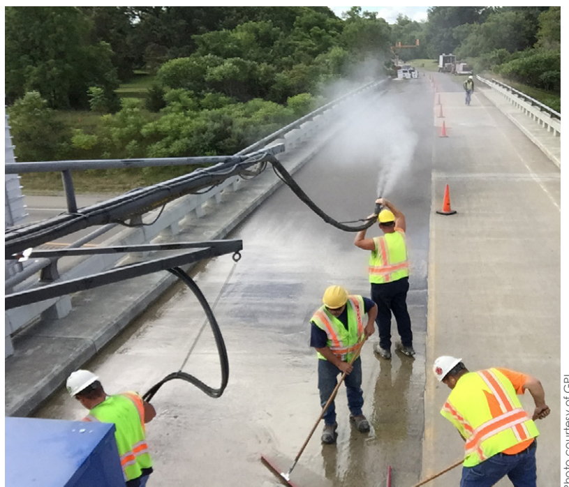
Figure 4. Broadcasting aggregate on sealer.
