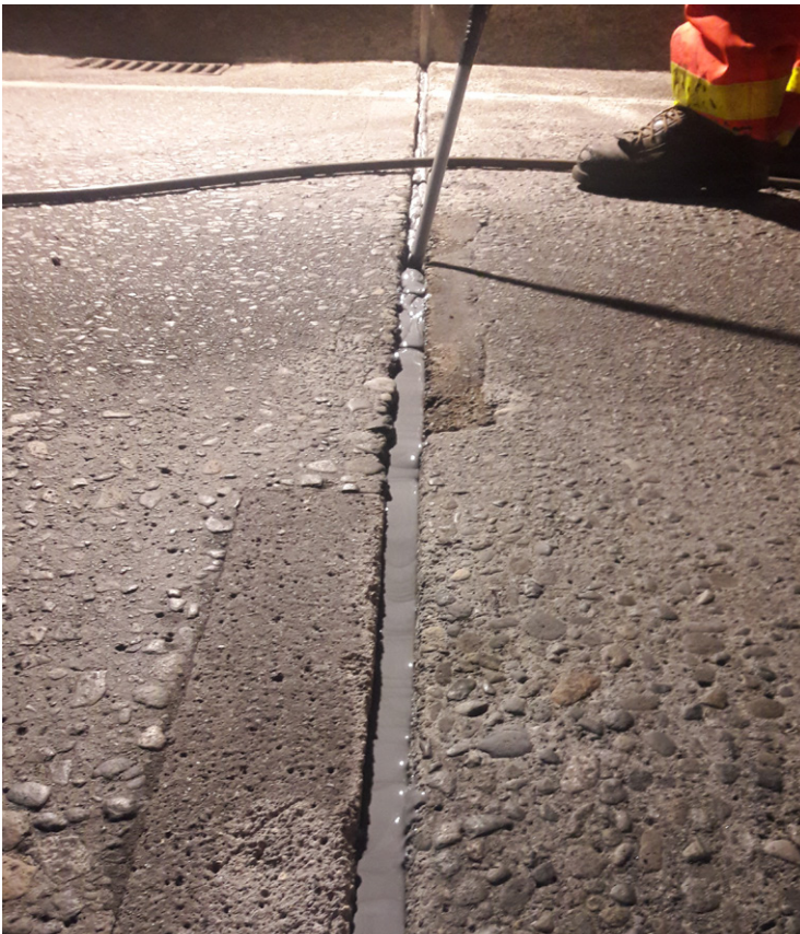
Figure 9. Joint seal replacement.
