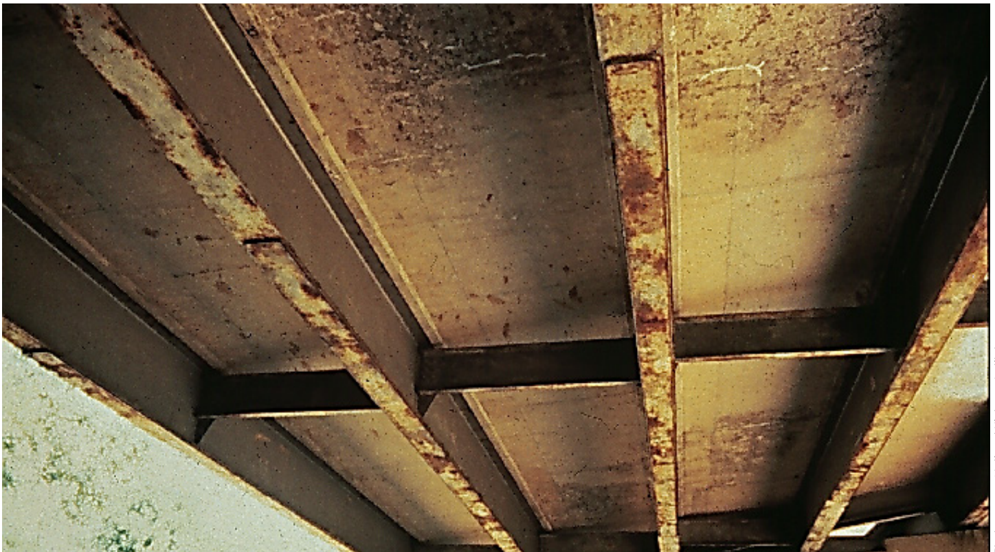
Figure 13. Diaphragms in straight steel bridges are not NBEs because they are not primary load-carrying elements, but they can be added as an ADE.
