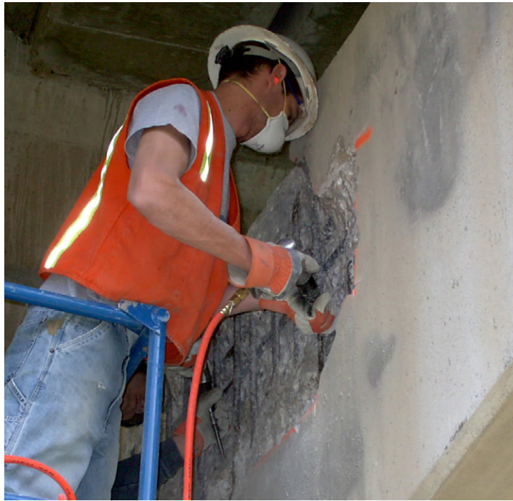
Figure 6. Substructure repair.
