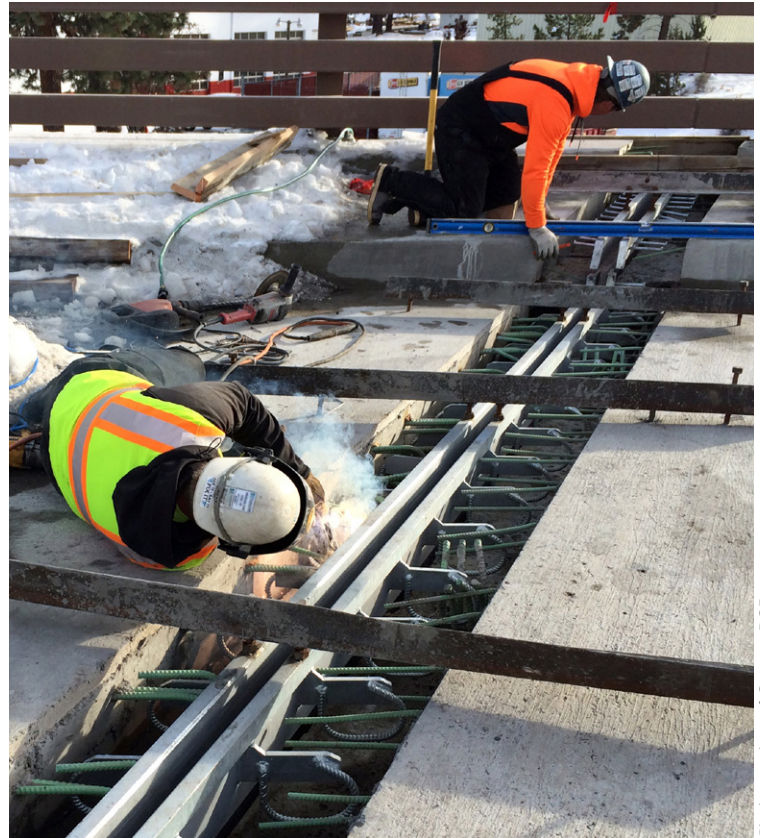
Figure 8. Joint replacement.
