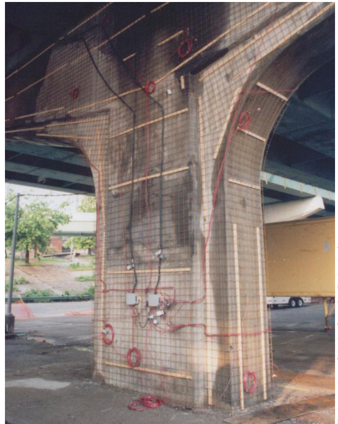
Figure 10. Pier being prepared for ECE treatment.
