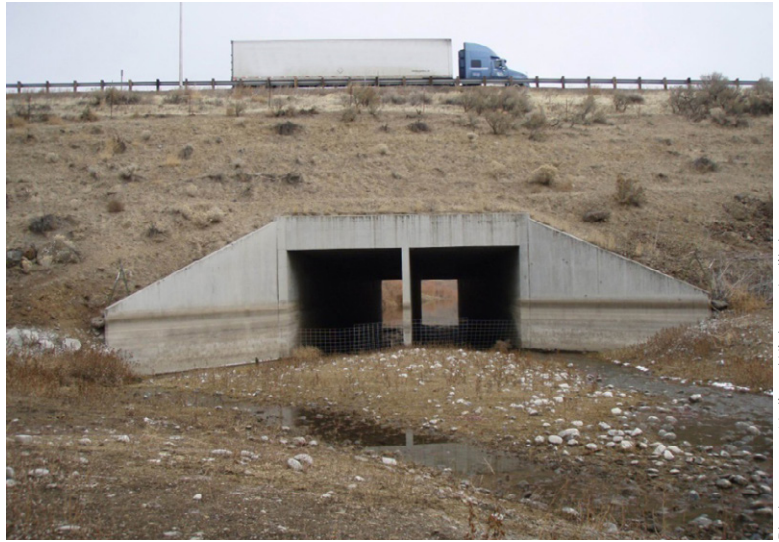
Figure 12. Culvert coded as Item 62. Superstructure and substructure coded as N.
