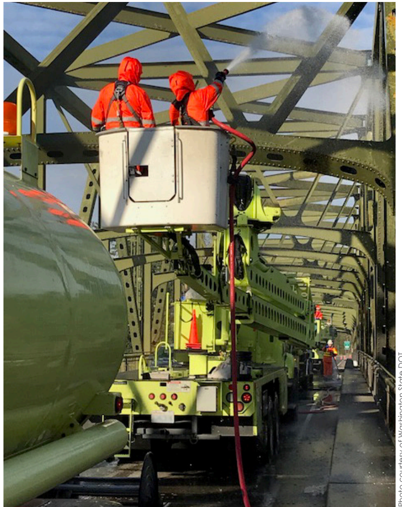
Figure 3. Bridge washing.
