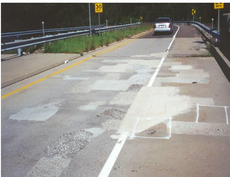
Figure 5. Deck showing halo effect.
