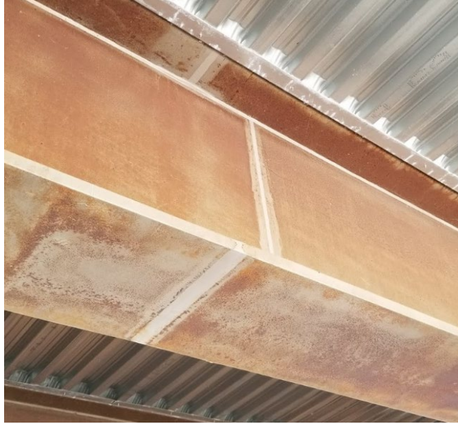
Figure 38. Photo. Steel plate girder with flange-to-web welds intersecting CJP groove welds in butt joints used to accomplish flange and web shop splices.
