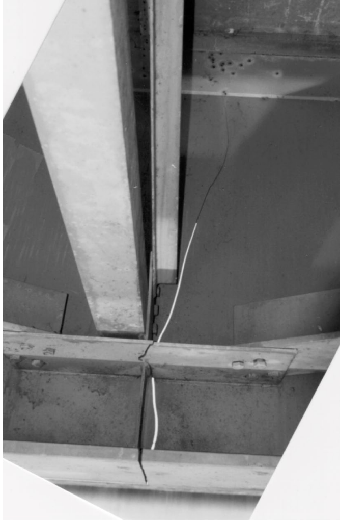
Figure 25. Photo. View of fracture in the outside plate girder of the I-64 Blue River Bridge.
