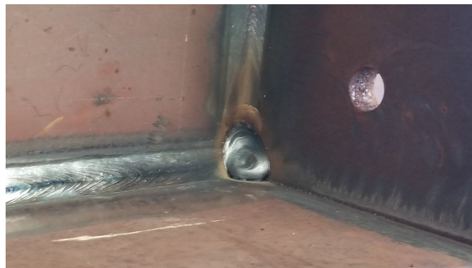
Figure 60. Photo. Transverse stiffener-to-web weld continuous into the corner at the intersection of the stiffener, web, and flange.
