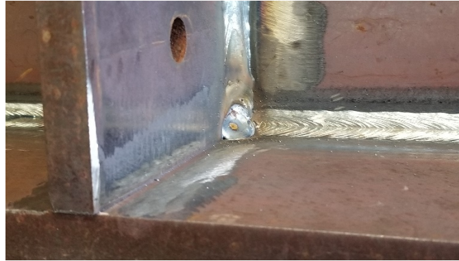
Figure 60. Photo. Transverse stiffener-to-web weld continuous into the corner at the intersection of the stiffener, web, and flange.
