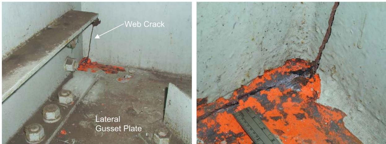
Figure 22. Photo. Fractured bottom flange of girder and arrested web fracture in the US 422 bridge. View of web on opposite side of lateral gusset connection.
