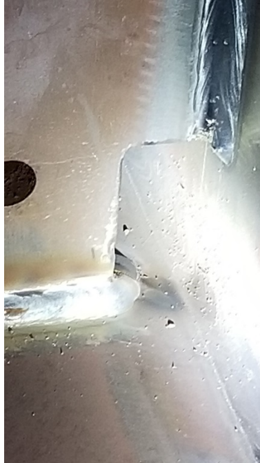
Figure 64. Photo. Transverse stiffener-to-flange weld completely wrapped around the base of a coped stiffener for sealing.
