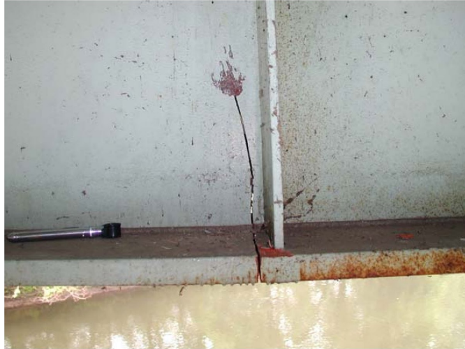
Figure 22. Photo. Fractured bottom flange of girder and arrested web fracture in the US 422 bridge. View of web on opposite side of lateral gusset connection.
