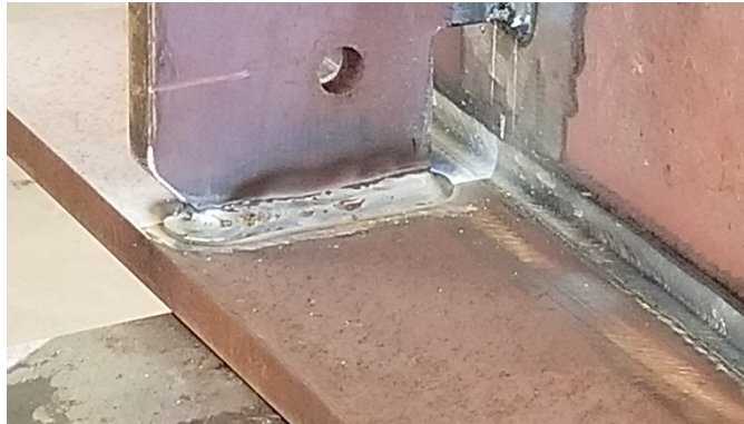
Figure 62. Photo. Transverse stiffener-to-flange weld completely wrapped around the base of a coped stiffener for sealing.
