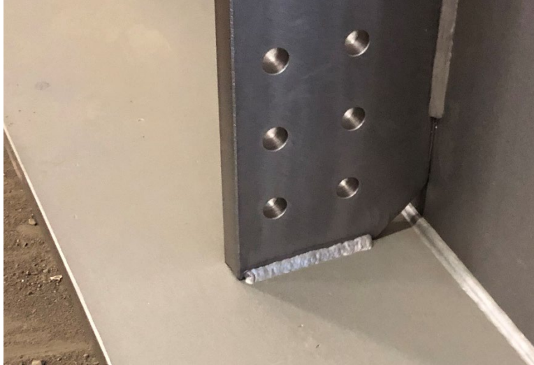
Figure 58. Photo. Transverse stiffener to a steel plate girder.
