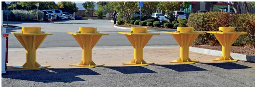
Figure 2. Photo. Passive entanglement barrier.
