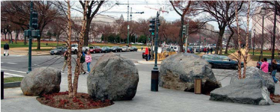
Figure 36. Photo. Large rocks integrated with bollards in recreational area.
