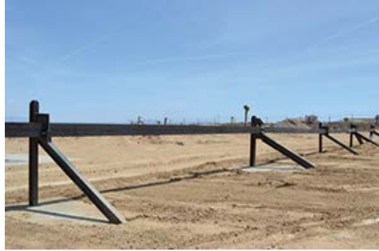
Figure 28. Photo. Post and Beam.
