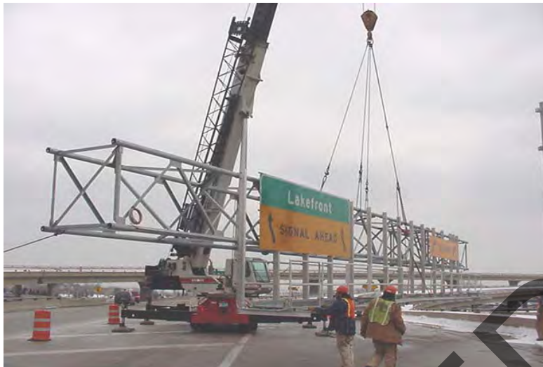
Figure 7. Assembled Truss Being Lifted Into Place.
