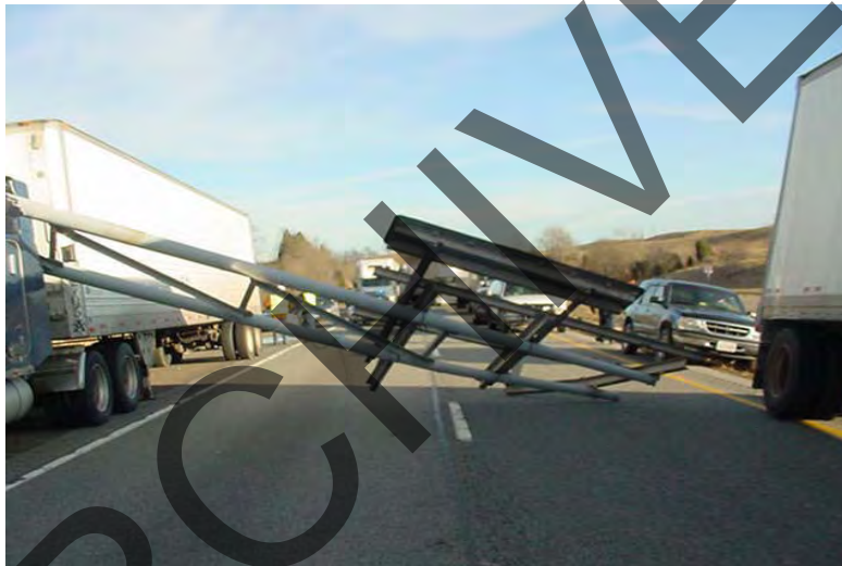
Figure 1. Cantilever Sign Structure Failure.
