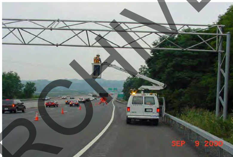
Figure 18. Bucket Truck-Most Common Way to Access Sign Structure.
