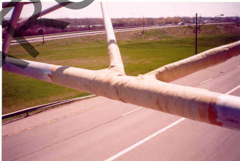
Figure 37. Repair of Truss Members Using FRP.
