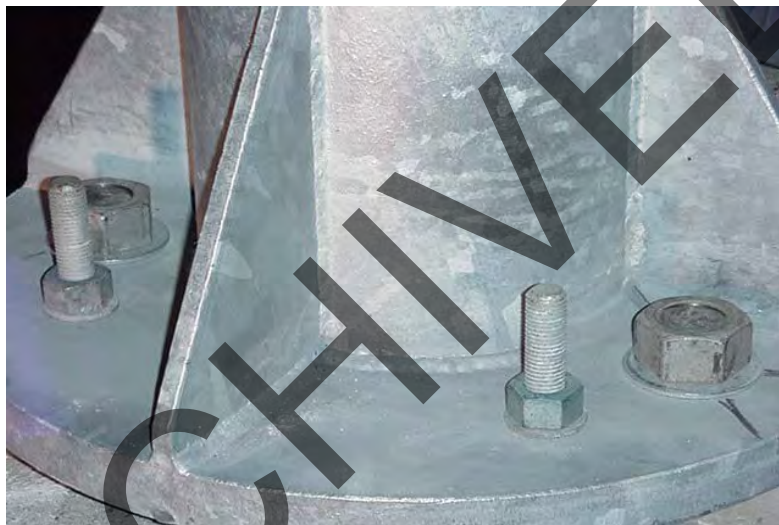
Figure 35. Base plate with Added Anchor Rods.
