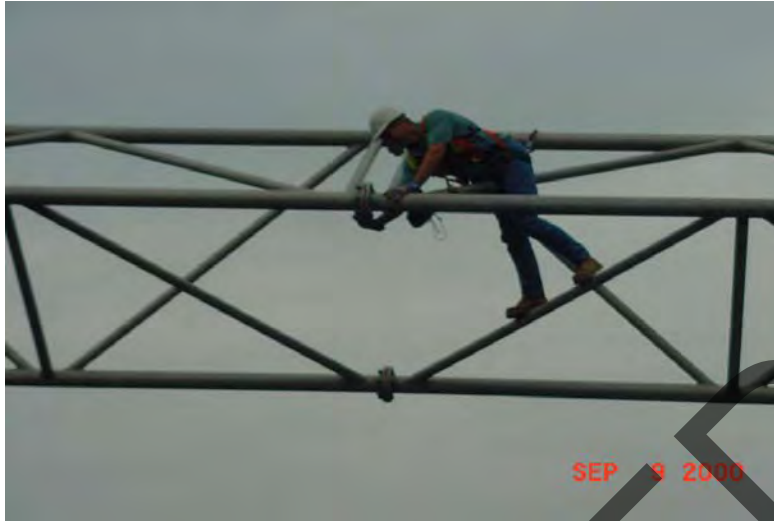
Figure 25. Hands on Inspection of Overhead Signs.
