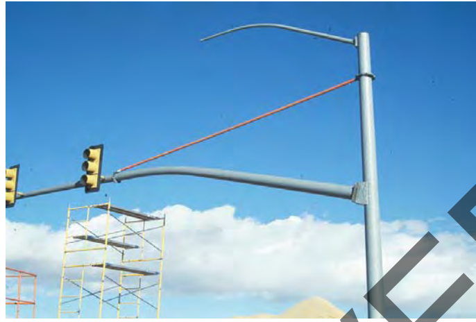
Figure 40. Wyoming Strand Damper.
