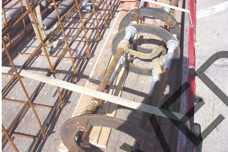
Figure 13. Four Anchor Rod Group in a Template. Note Top is Galvanized.
