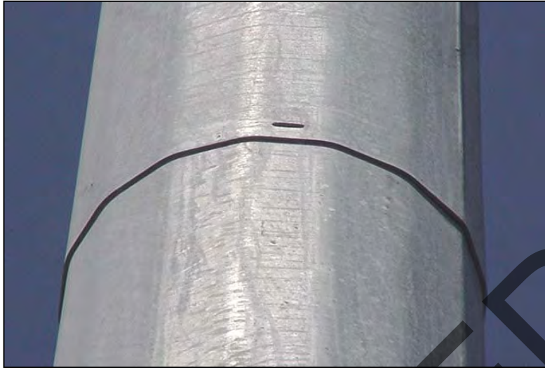
Figure 29. High Mast Pole Slip Joint.
