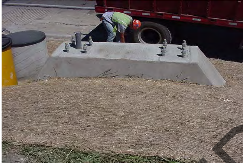
Figure 5. Foundation Ready for Structure Installation.
