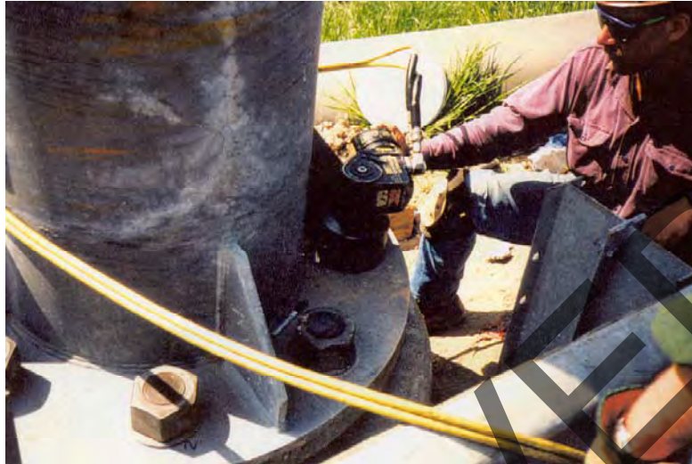
Figure 15. A Hydraulic Torque Wrench Tightening Anchor Rod Nuts to Achieve Needed Rotation.
