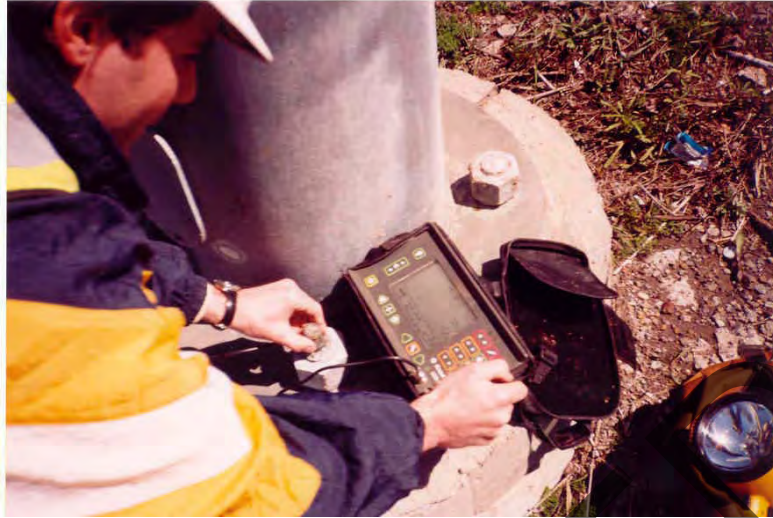
Figure 33. Ultrasonic Testing of Anchor Rods.
