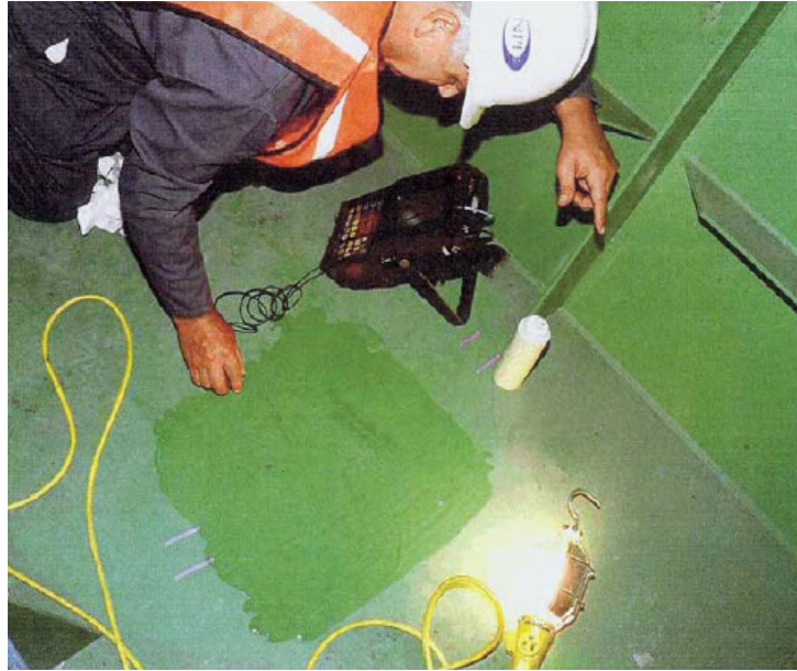
Figure 9.3.3.1-4 Ultrasonic testing of electro-slag welds.
