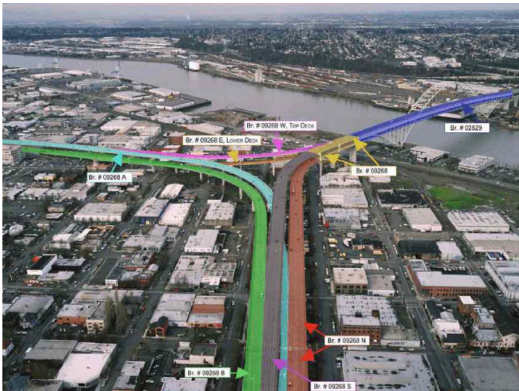
Figure 9.3.3.1-1 Fremont Bridge in Portland, Oregon.
