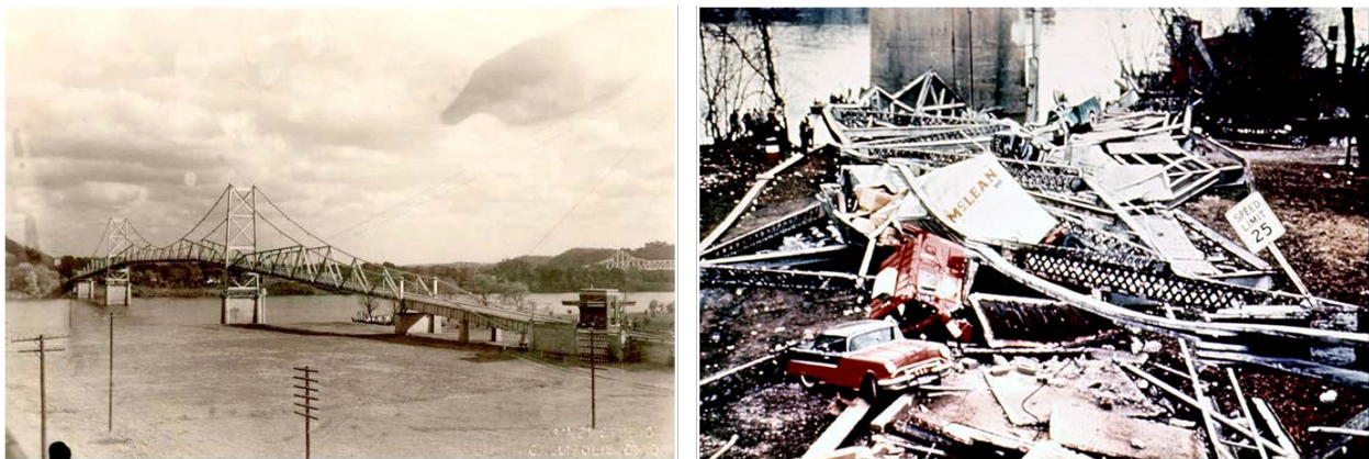
Figure 7.1-1 Point Pleasant Bridge before and after its collapse.
