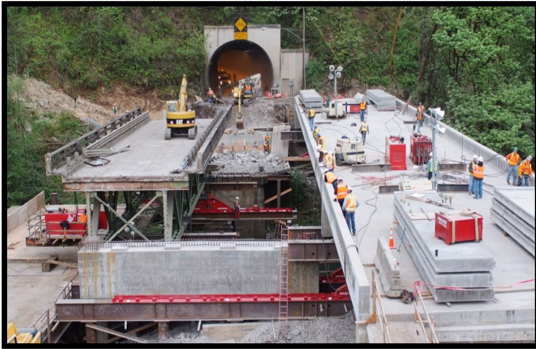
Figure 3-2 SIBC with Large Site Constraints at the OR-38 Bridge Project, Oregon
