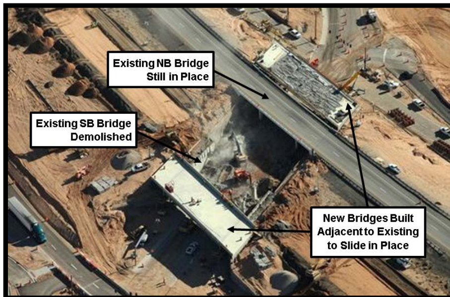
Figure 1-1 Overhead View of the West Mesquite SIBC Project, Nevada
