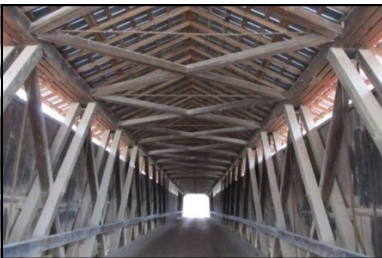
Pine Bluff Bridge, IN (Howe Truss)
