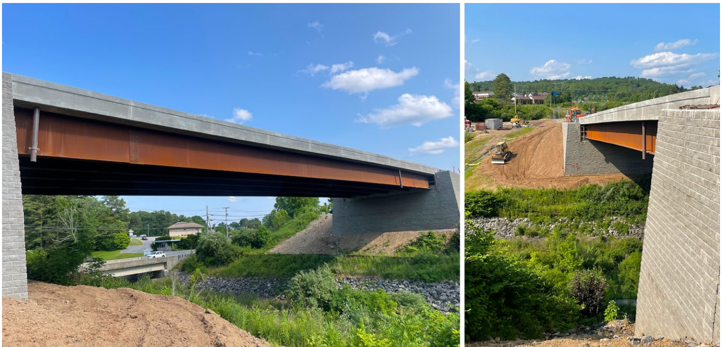
West Virginia used the geosynthetic reinforced soil-integrated bridge system (GRS-IBS) on a 190-foot span.
