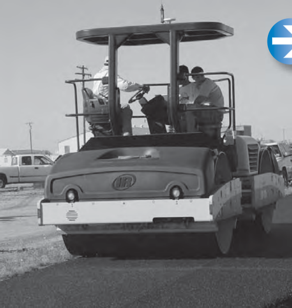
The intelligent asphalt compaction analyzer is mounted on compaction equipment to provide real-time data so problems can be fixed during the paving process.
