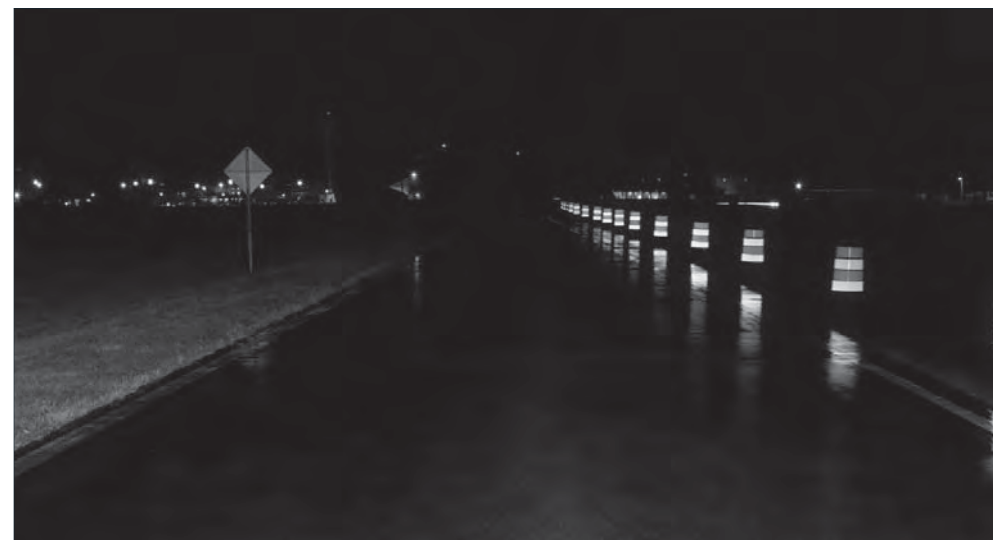
The all-weather pavement marking system (top photo) makes it easier for drivers to navigate wet roads than conventional markings (bottom photo).
