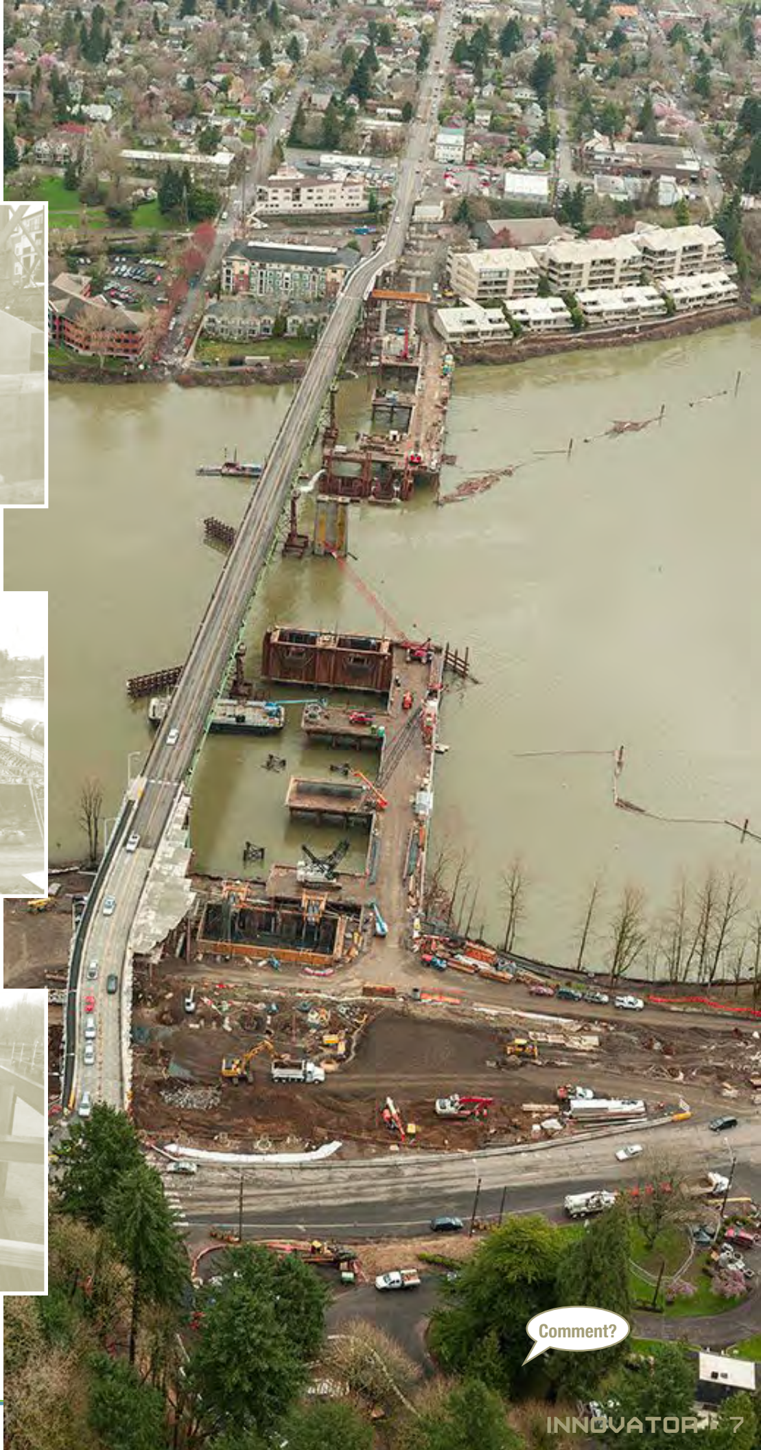
Foundation work is under way for the new bridge.
