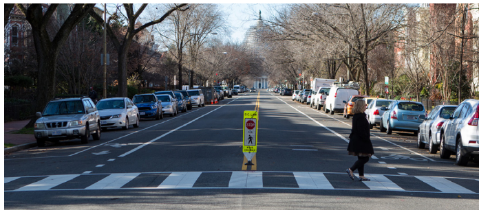
Crosswalk visibility enhancements such as high-visibility markings and in-street signs help make crosswalks and pedestrians more visible.
