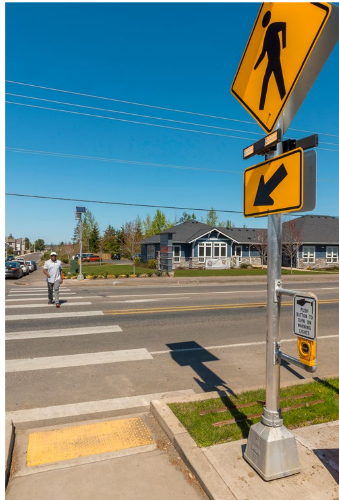
Oregon is installing more rectangular rapid flashing beacons to help alert drivers to the presence of pedestrians.
