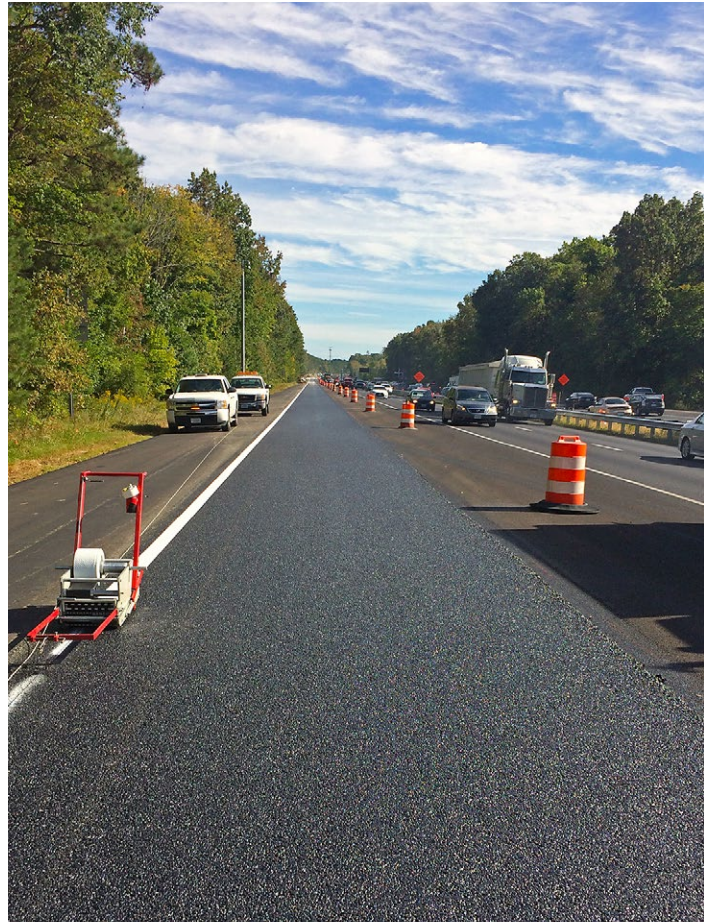
In 2017, Virginia DOT placed SMA HiMA in the right lane and kept conventional SMA in the left lane as a control for a field evaluation.
