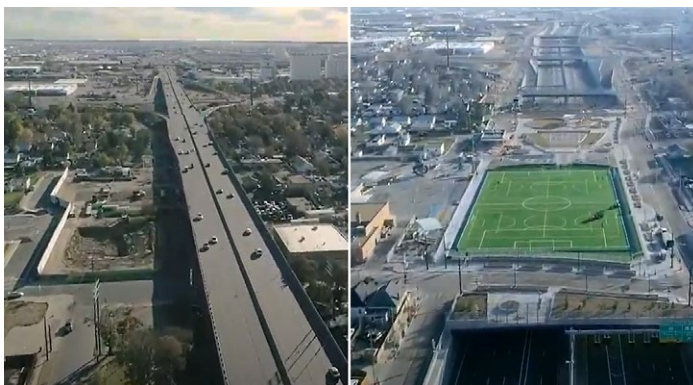
The Central 70 Project removed an aging viaduct (shown in photo on left), lowered the interstate, and built a new 4-acre cover park (shown in photo on right) for the surrounding community.
