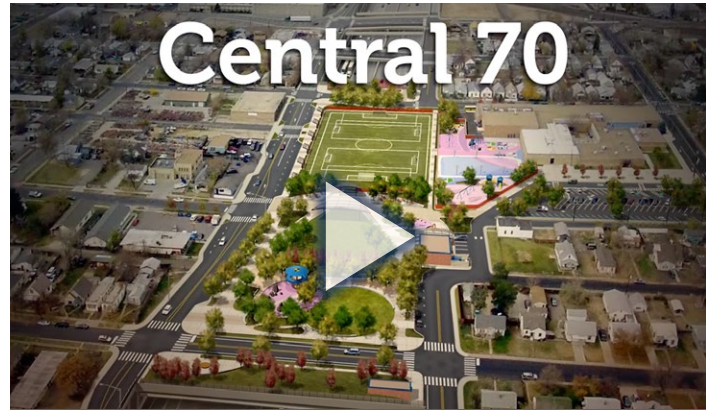
CDOT used videos to supplement public meetings and other outreach for residents in the Central 70 project area.
