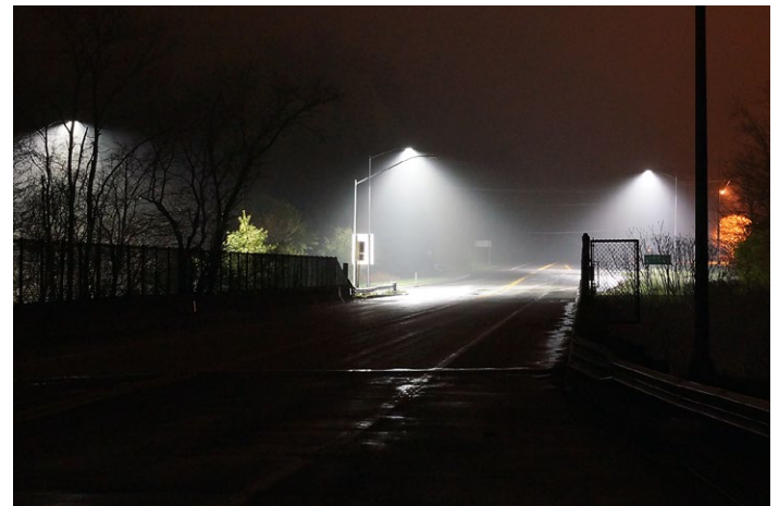
Enhanced lighting at a rural intersection.
