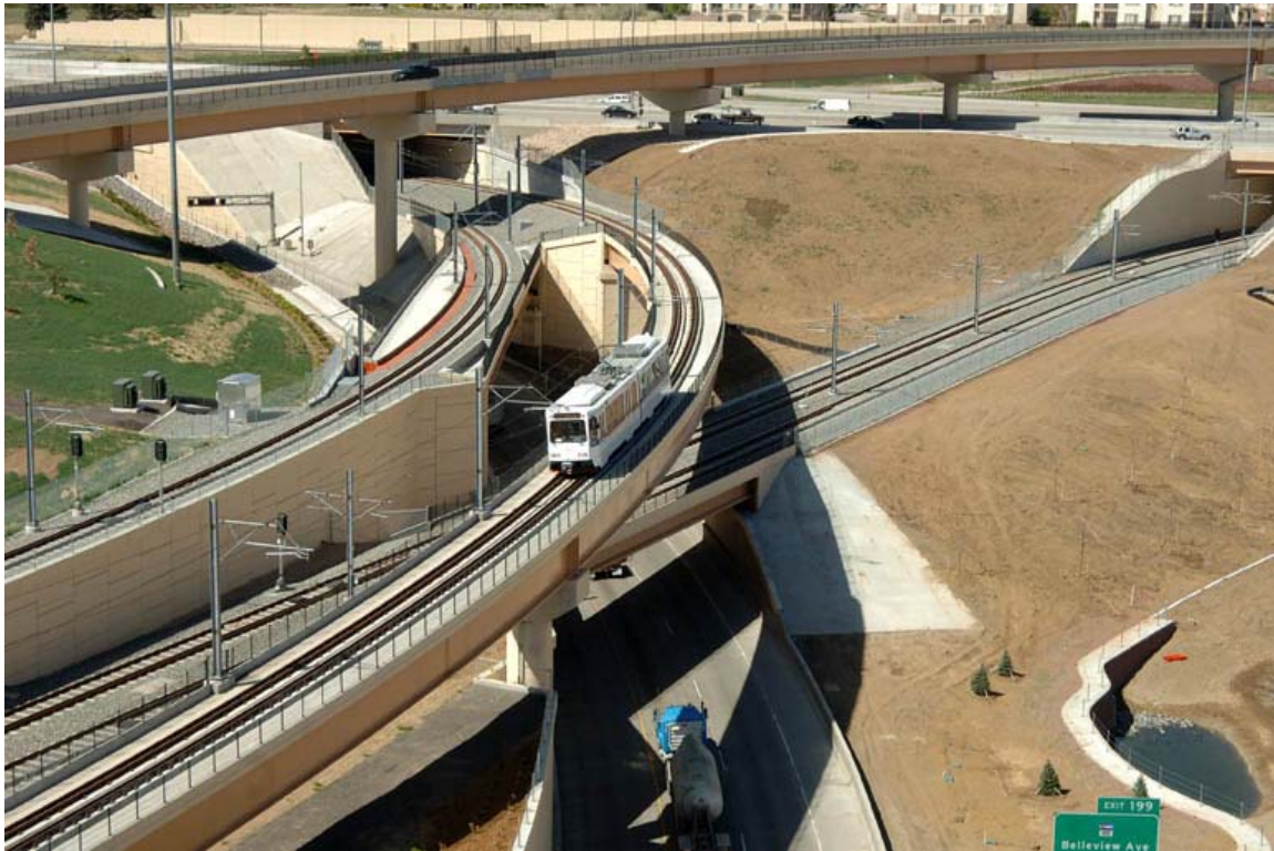
[An operational view of T-REX, showing the LRT and highway systems]
