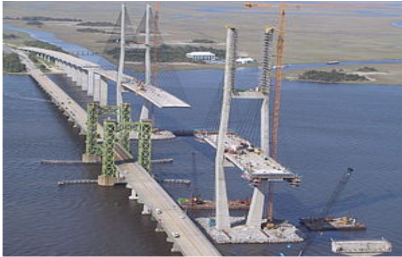
Sidney Lanier Bridge, Brunswick
