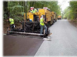
Photo Courtesy of Sealcoating, Inc.
