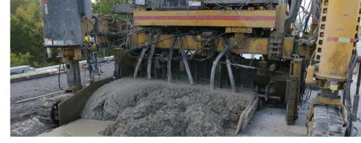
Two-lift concrete paving, as shown here, uses a higher percentage of recycled or marginal aggregate in a thicker bottom layer, while reserving more durable material for the thinner surface layer, thereby improving the sustainability of the pavement without compromising performance. Source: APTech.
