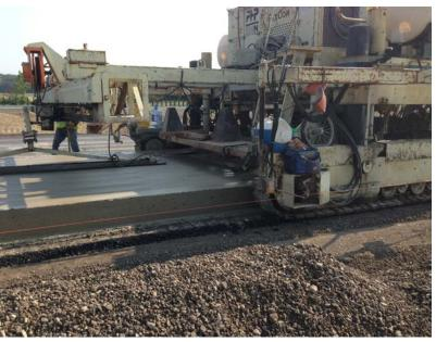
A new materials specification is expected to improve the durability and longevity of the Nation's concrete pavements. Source: APTech.
