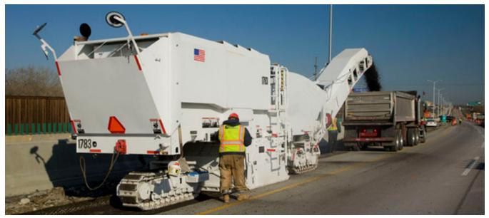
A milling machine is removing layers of asphalt pavement to generate recycled asphalt pavement, or RAP, as part of a rehabilitation project. Source: Astec Industries.
