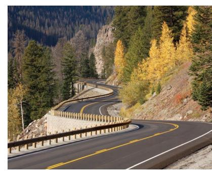
Warm-mix asphalt, which was used when paving this stretch of scenic roadway in Yellowstone National Park, is an innovation that improves the sustainability of pavements by requiring about 20 percent less energy to produce.
