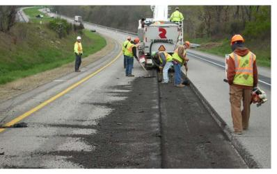
A crew is repairing a longitudinal joint in Pennsylvania using a mill and fill patching process along the full length of the pavement. *Source: PennDOT.*
