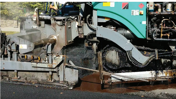
All States Materials Group Figure 7. Ultrathin bonded wearing course
