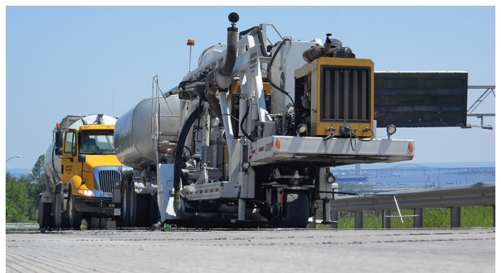
International Grooving and Grinding Association Figure 12. Diamond grinding
