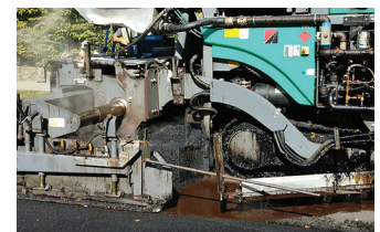
All States Materials Group Figure 4. Ultrathin bonded wearing course
