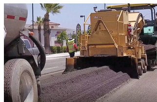
Pavement Recycling Systems Figure 3. Cold in-place recycling
