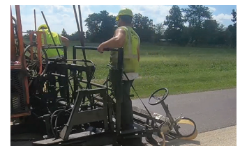
Strawser Construction Inc. Figure 6. Cape sealing
