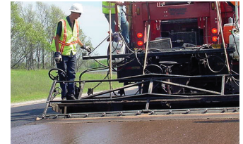
National Center for Pavement Preservation Figure 2. Micro surfacing
