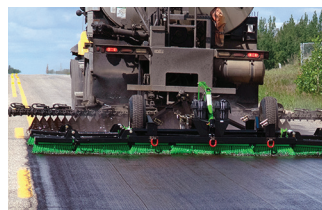
Saskatchewan Ministry of Highways and Infrastructure Figure 5. Scrub sealing
