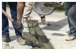
ACPA Figure 7. Partial-depth repair
