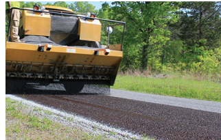
Slurry Pavers, Inc. Figure 1. Chip sealing
