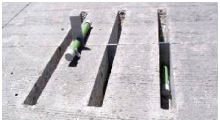
ACPA Figure 6. Dowel bar retrofit
