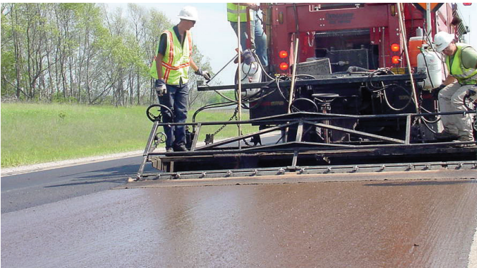
National Center for Pavement Preservation Figure 2. Micro surfacing
