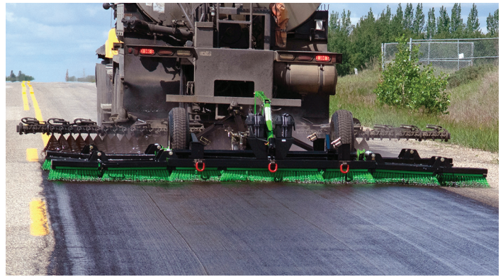
Saskatchewan Ministry of Highways and Infrastructure Figure 4. Scrub sealing
