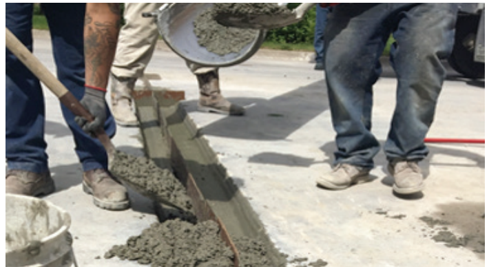
ACPA Figure 5. Partial-depth repair
