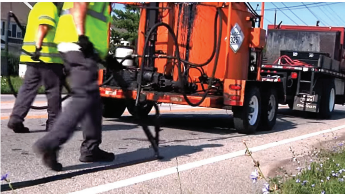
National Center for Pavement Preservation Figure 1. Crack sealing
