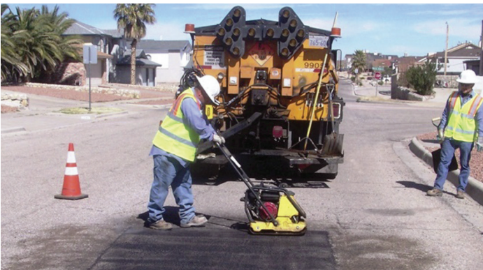
City of El Paso Figure 3. Asphalt patching
