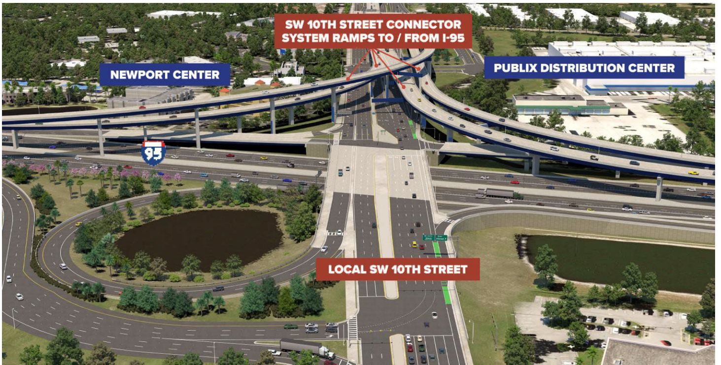
Figure 3: SW 10 th St Connector at I-95 Interchange reconstruction
