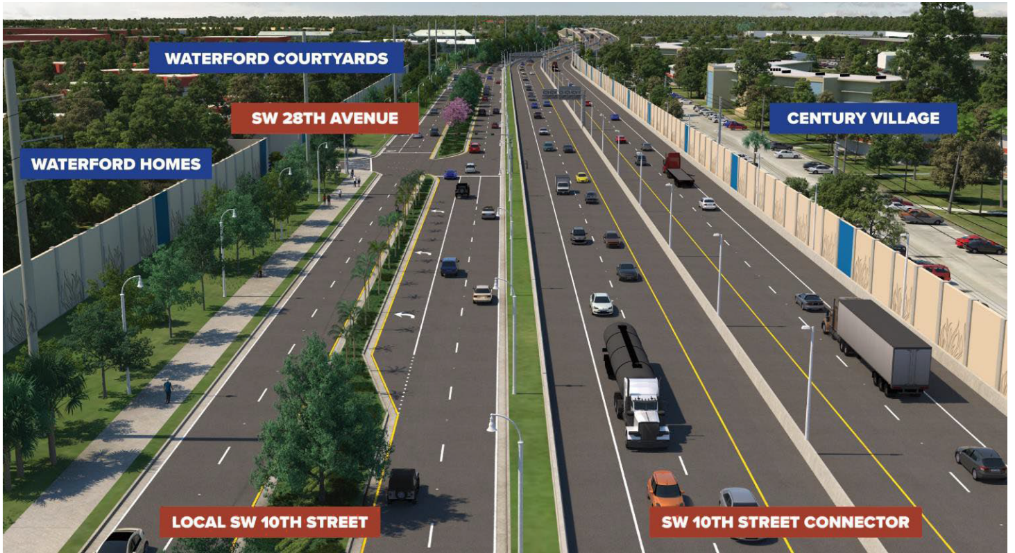
Figure 2: SW 10 th St Connector and Local SW 10 th St facilities sharing existing R/W
