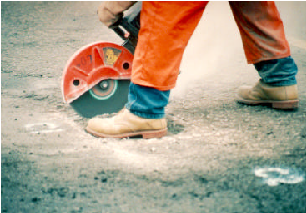
Figure 3. Semi-permanent procedure—straightening edges using hand-held pavement saw.
