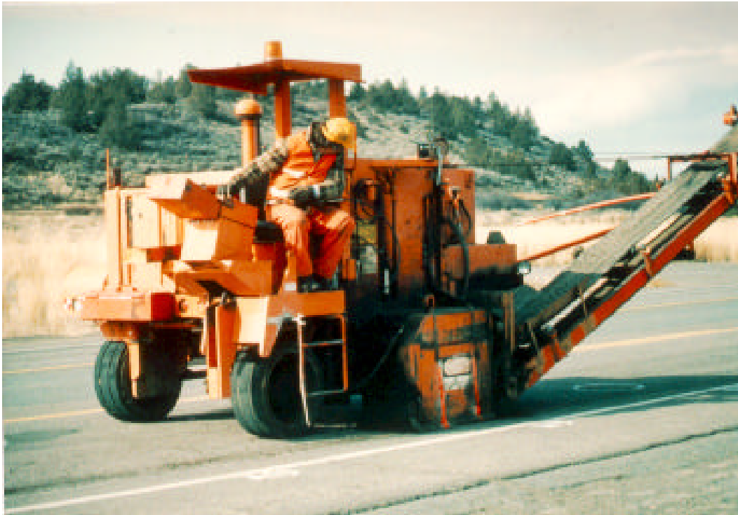
Figure 4. Semi-permanent procedure—straightening edges using cold-milling machine.
