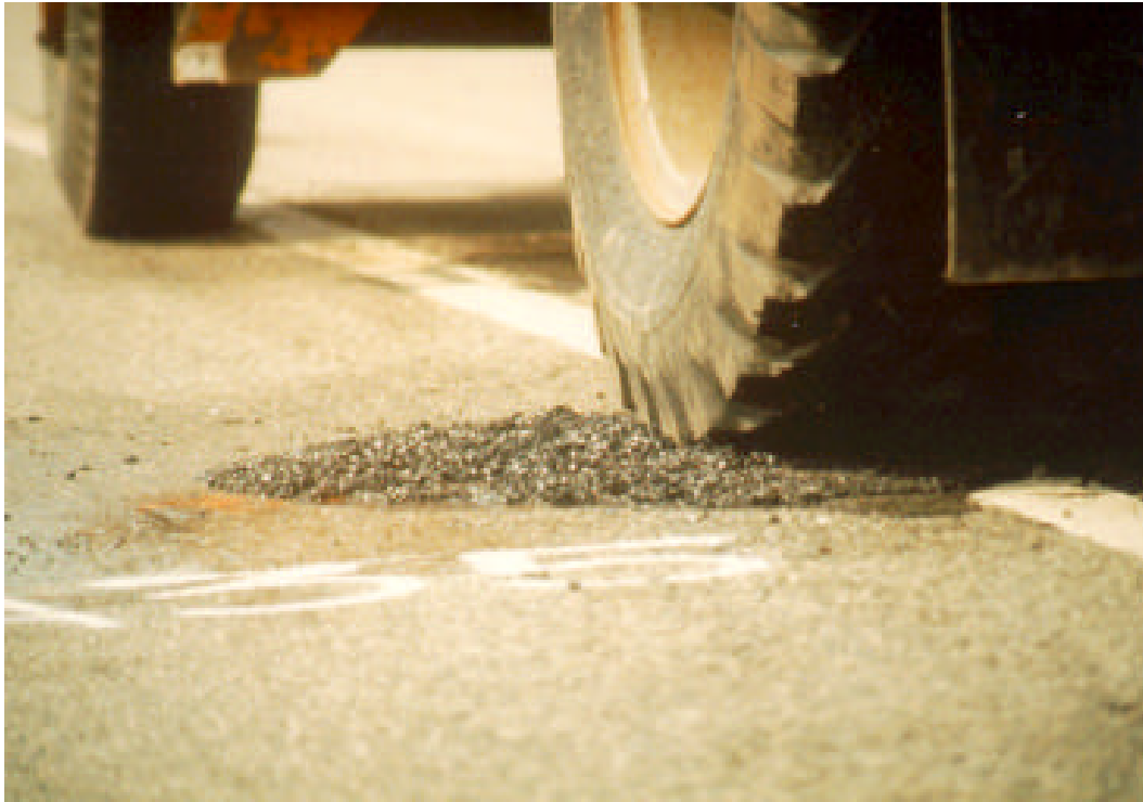
Figure 2. Throw-and-roll procedure—compaction of patch.
