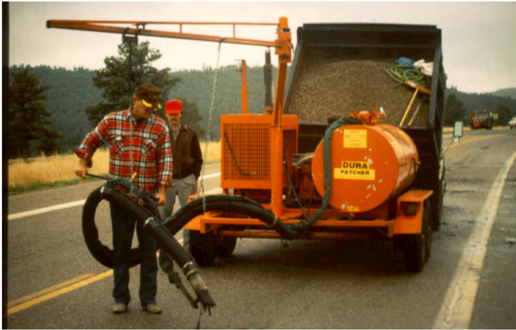
Figure 7. Spray-injection device—truck and trailer unit.
