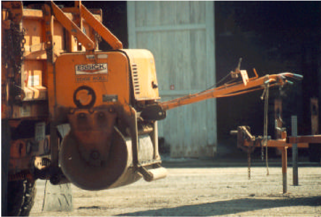
Figure 6. Semi-permanent procedure—single-drum vibratory roller used for compaction.
