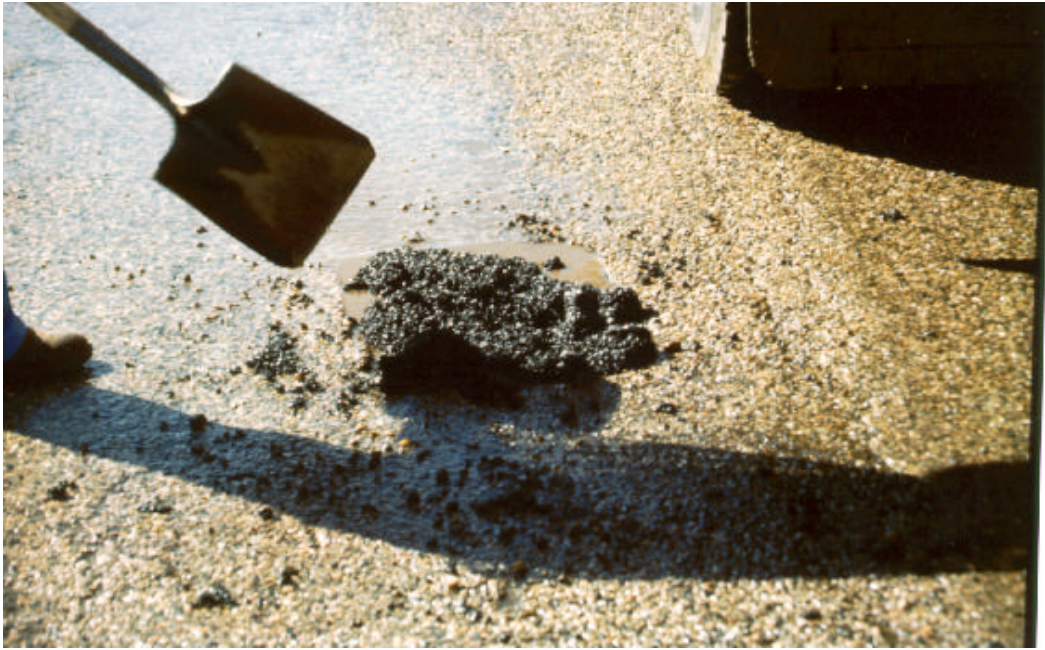
Figure 1. Throw-and-roll procedure—material placement.
