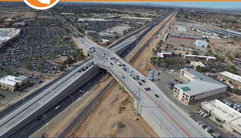
Figure 1: Newly constructed US-60/Bell Road Interchange in Surprise, Arizona (Photo Credit: City of Surprise)
