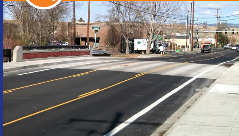
Figure 2: Recently reconstructed Ochoco Creek Bridge in Prineville, Oregon (Photo Credit: Oregon Department of Transportation)
