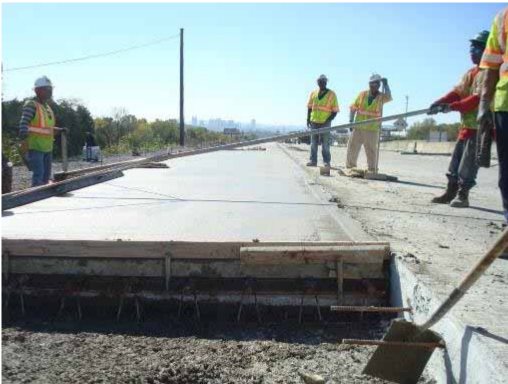
Photo E-44. Finishing pavement at Day 2 header.
