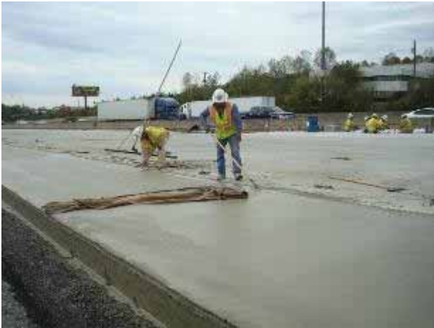
a. Maintaining longitudinal joint.
