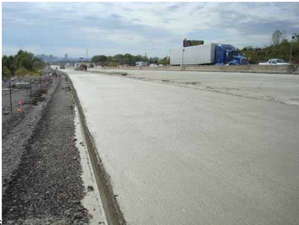
Photo E-30. Shoulder edge line after second edge slump correction effort.
