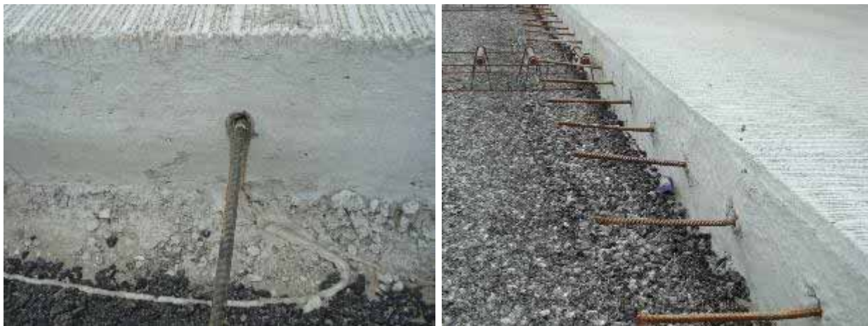
Figure 5. Tie bar placement.
