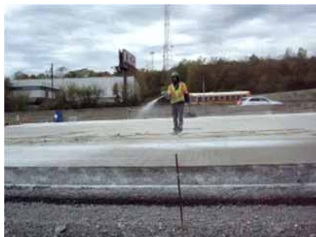
b. "Hand" spraying curing compound.
