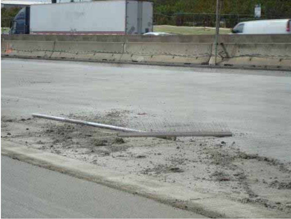
Photo E-49. Rake used for applying transverse tining.
