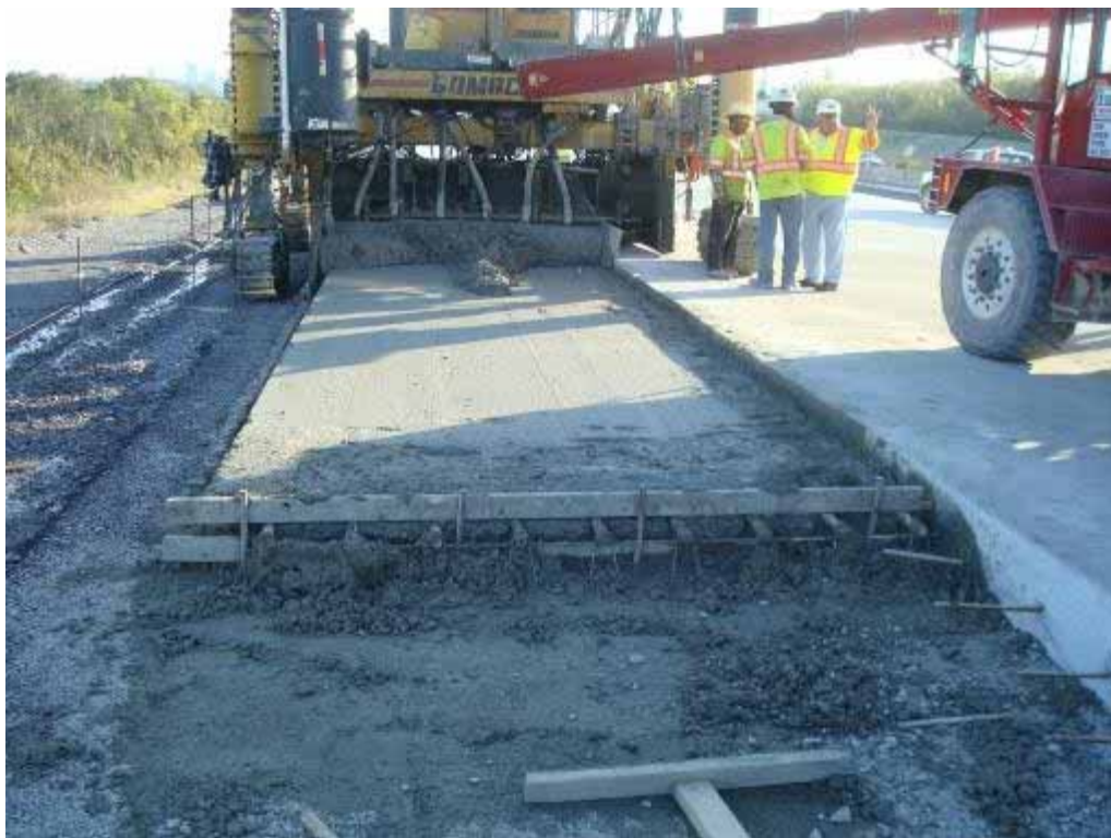
Photo E-36. Day 1 header, just prior to top lift placement.
