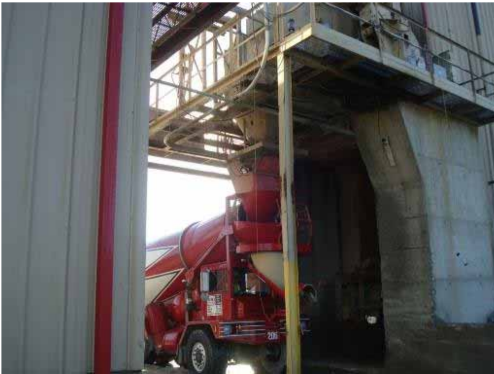
Photo E-8. Loading front-discharge drum truck with top lift concrete.
