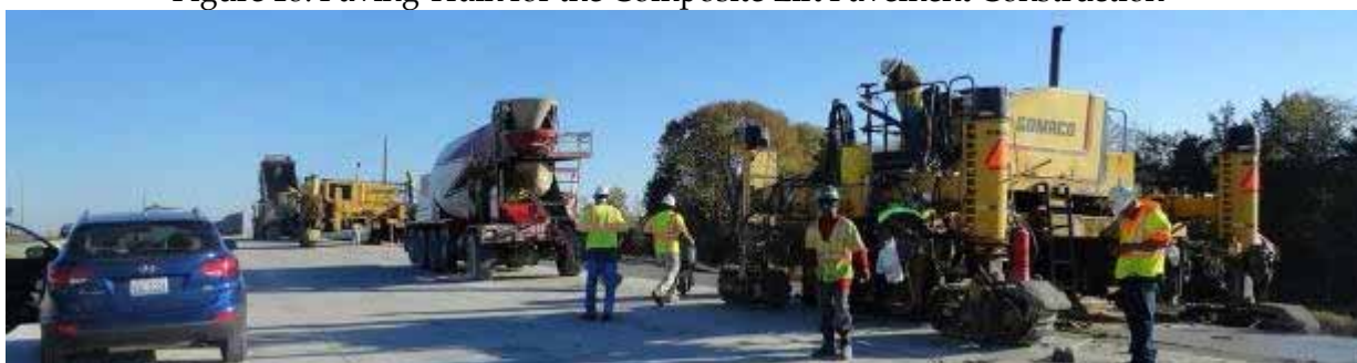
Figure 19: Paving Train for the Composite Lift Pavement Construction
