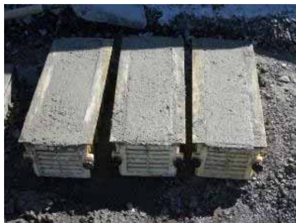
f. Beam preparation.
