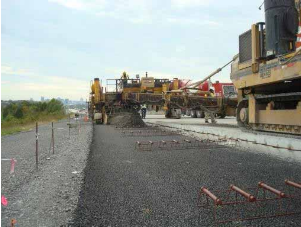
Photo E-15. Bottom lift paving, viewed from ahead of paver.
