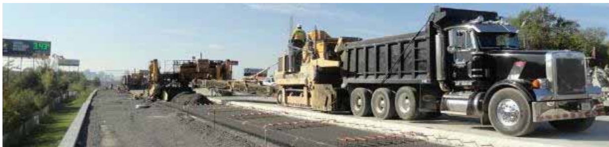
Figure 18: Paving Train for the Composite Lift Pavement Construction
