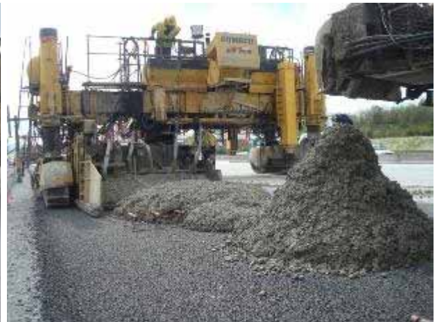
d. Mix placement and paver.
