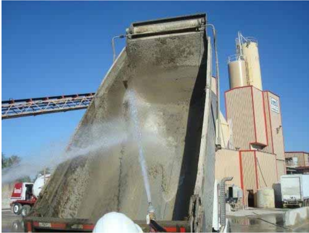
Photo E-11. Washing out dump truck at IMI ready-mix facility.
