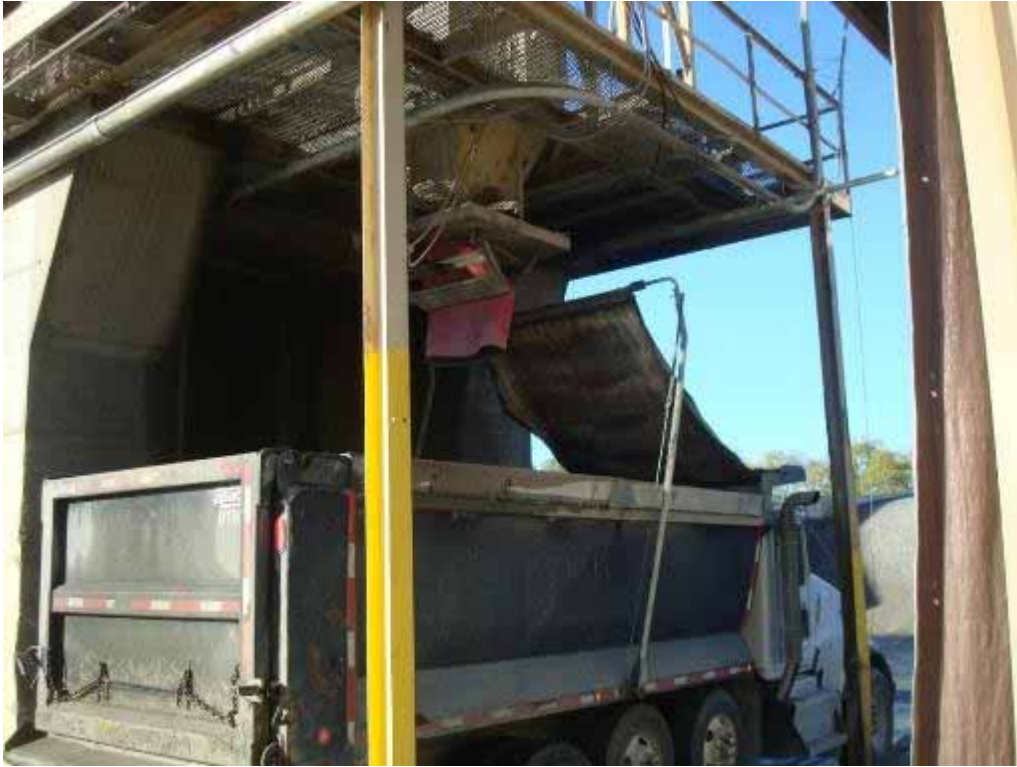
Photo E-7. Loading dump truck with bottom lift concrete mix.
