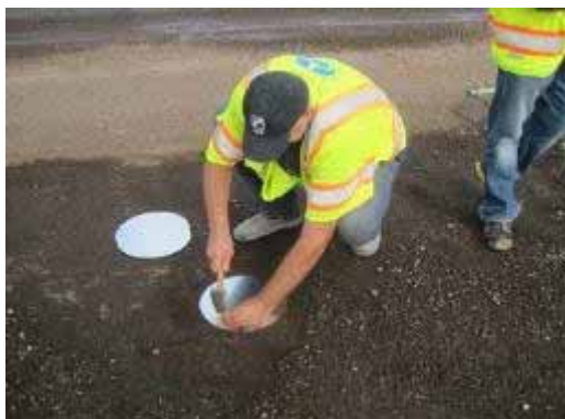
Figure 49: MCL staff Placing a Metal Target on the Base
