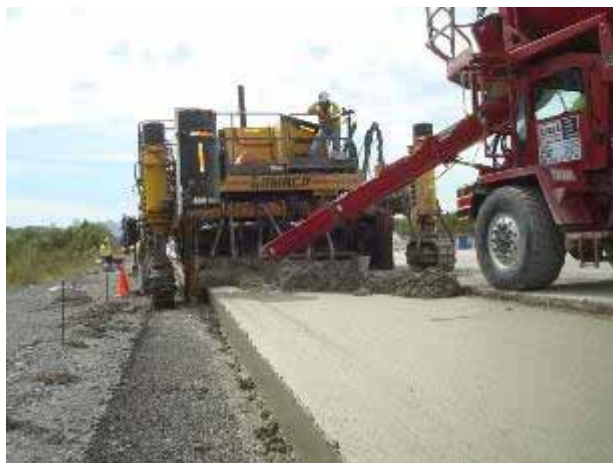
b. Mix delivery and paver.
