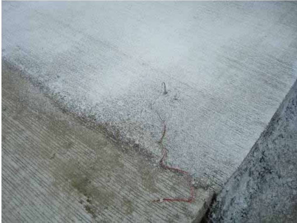
Photo E-55. Thermocouple/maturity sensor installation at south end of project.
