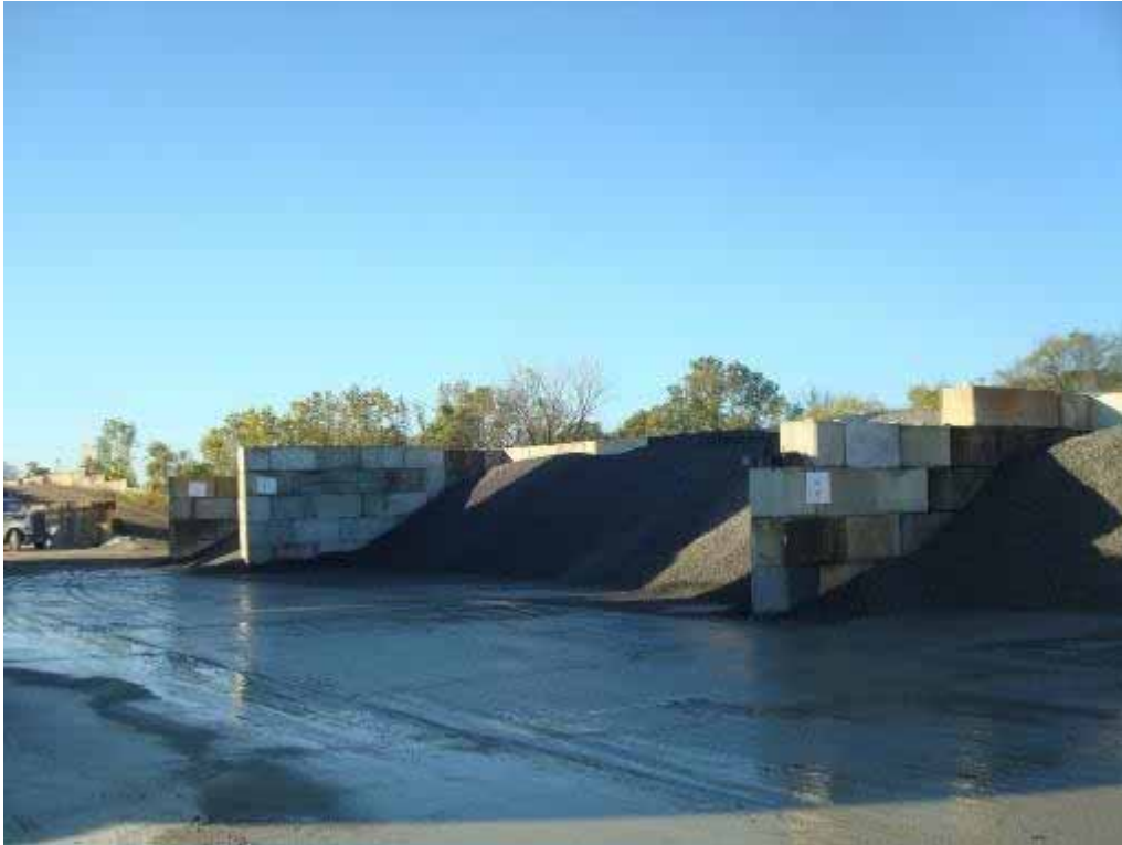
Photo E-5. Aggregate storage bins at IMI ready-mix.
