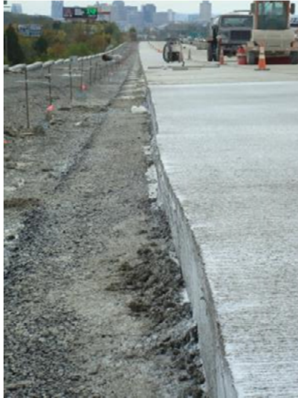
Photo E-33. Edge blowout #2 after repair.
