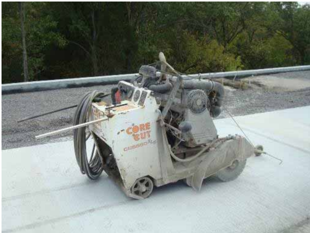
Photo E-56. Saw used for cutting transverse joints.
