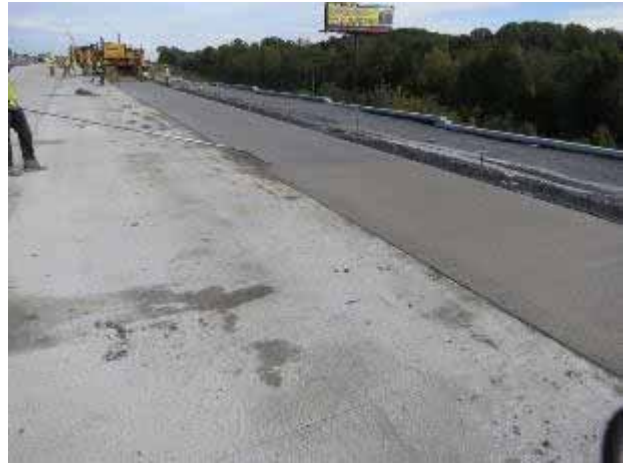
b. Concrete tining.
