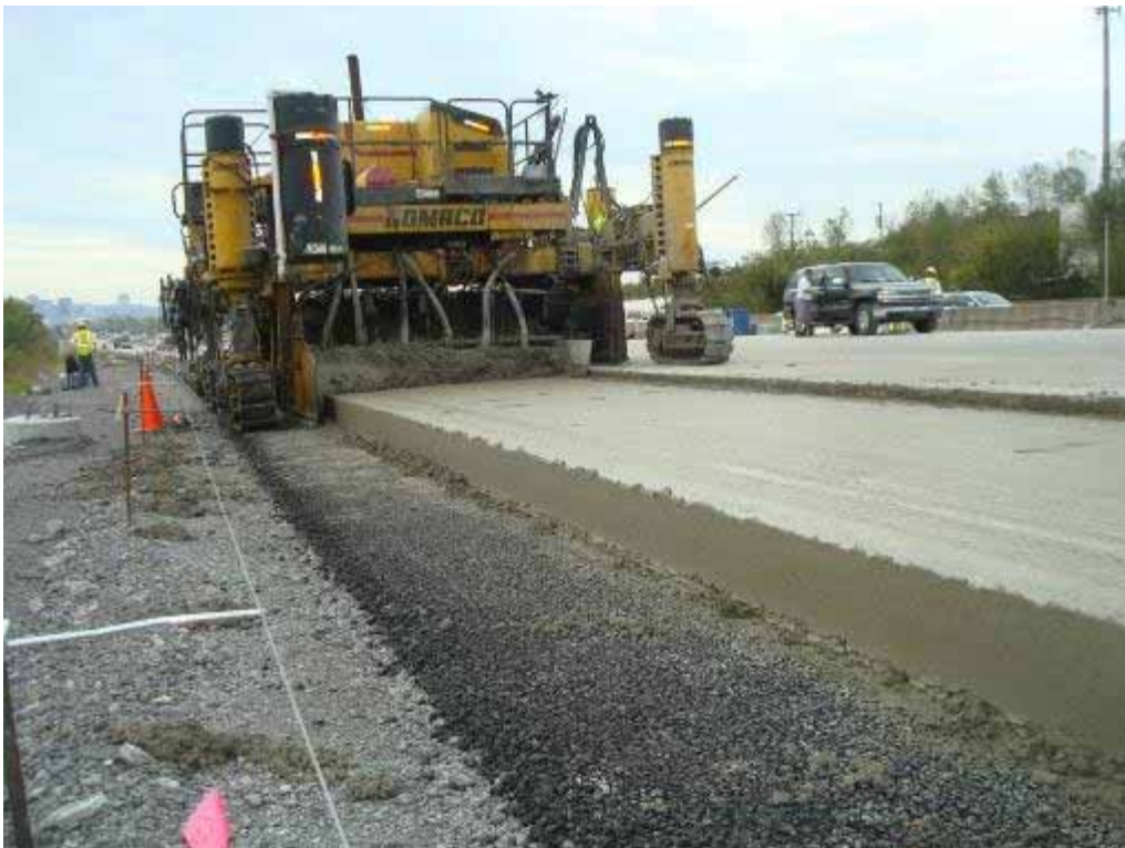
Photo E-18. Bottom lift paving, viewed from behind paver.
