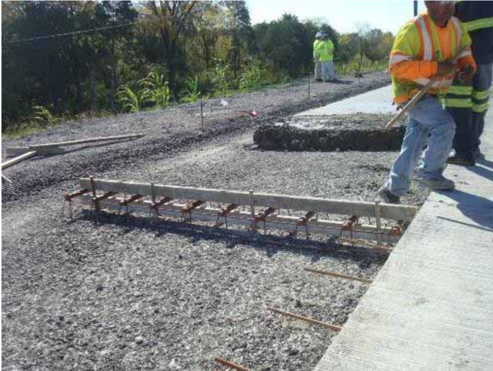
Photo E-43. Construction of Day 2 header.
