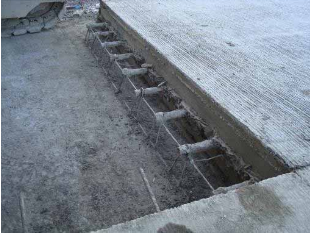
Photo E-37. Day 1 header after placement of both lifts.
