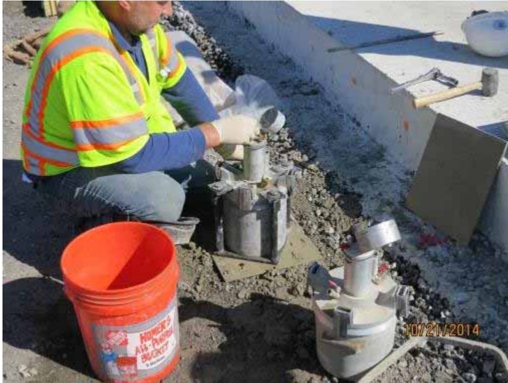
Photo E-47. Testing concrete using Super Air Meter (SAM).
