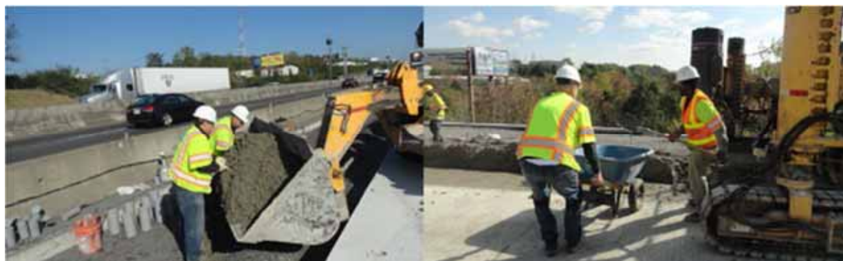
Figure 20: Sampling on the Grade
