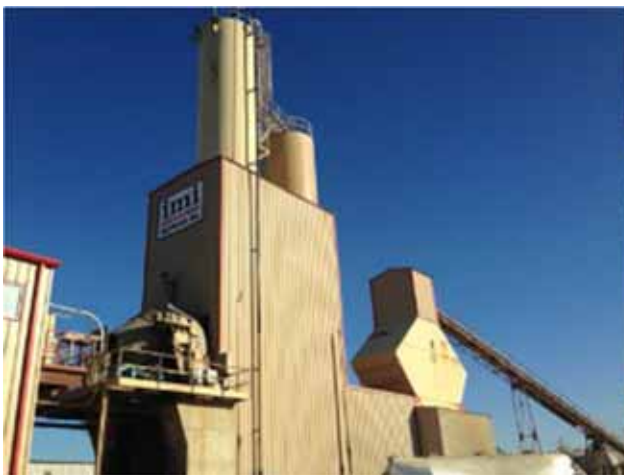
Figure 3: Concrete Batch Plant
