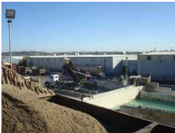
d. Wash water recycling facilities.
