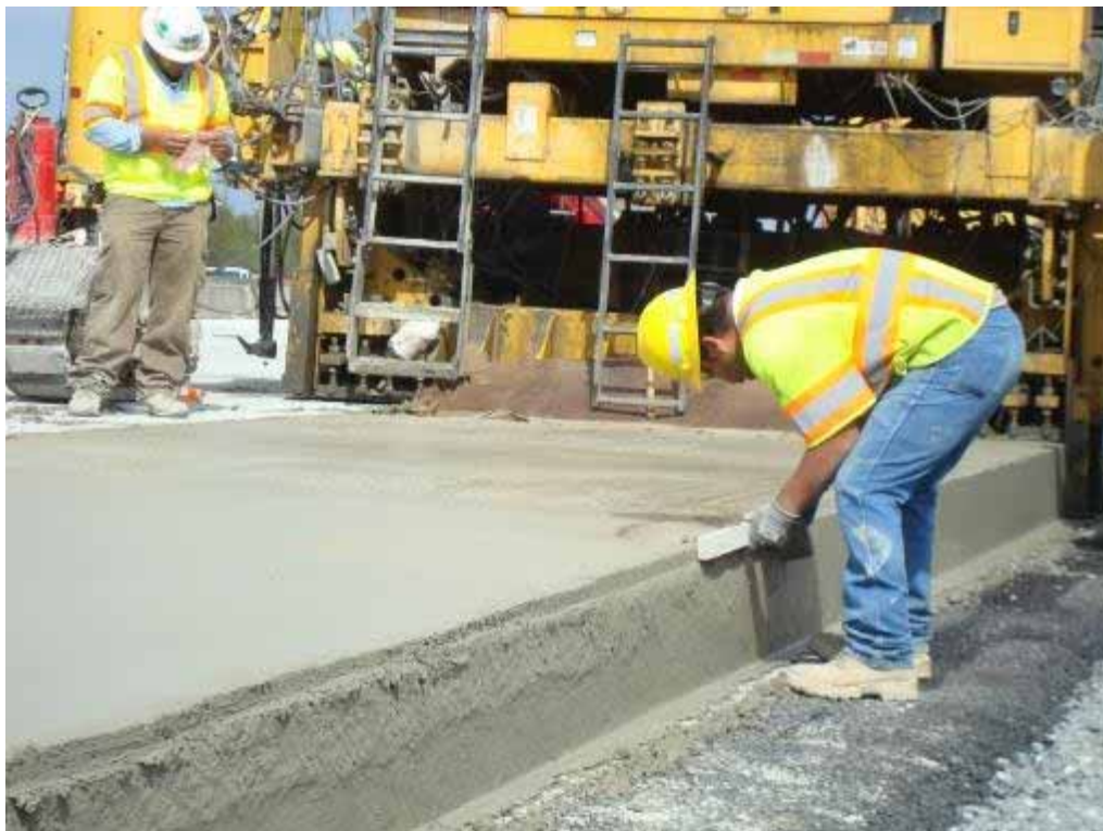
Photo E-28. Workers attempting to correct second lift edge slump.
