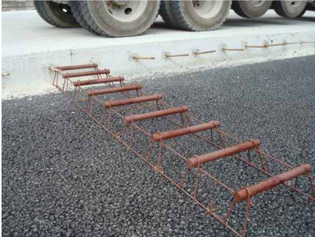
Photo E-3. Dowel basket anchored to asphalt-treated permeable base.
