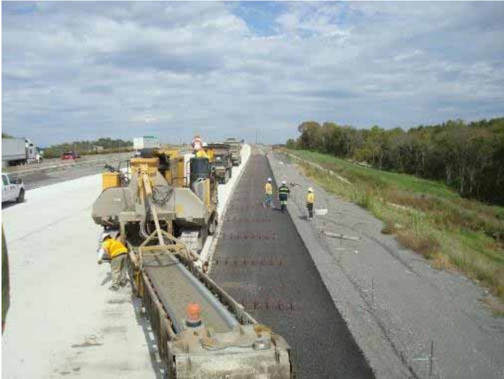
Photo E-17. View from top of first lift paver, looking ahead.
