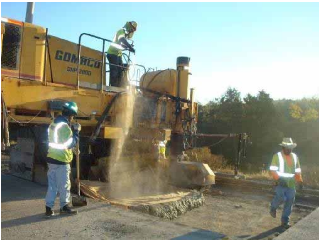
Photo E-38. Start of Day 2 paving, bottom lift.
