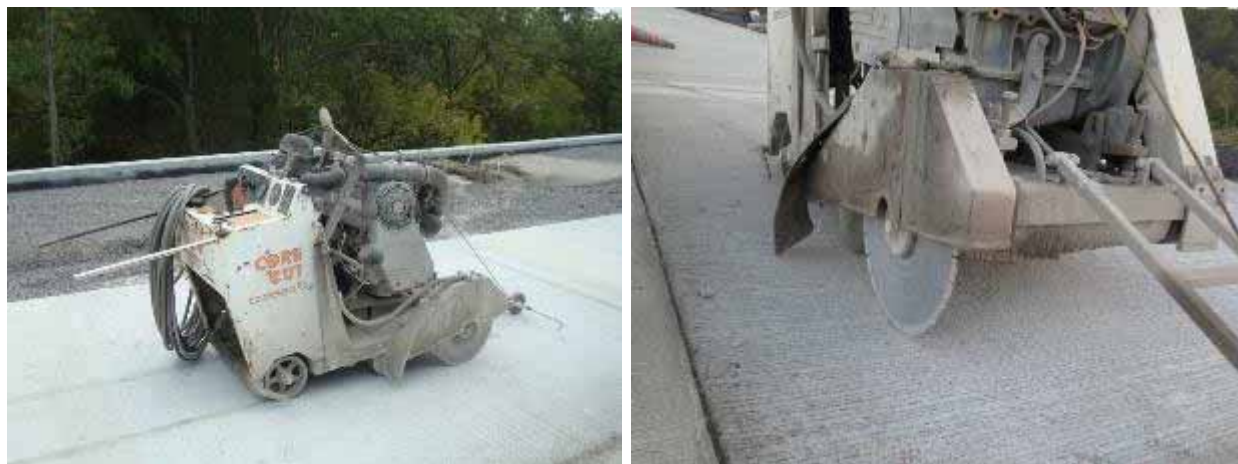
Figure 11. Transverse joint and saw.
