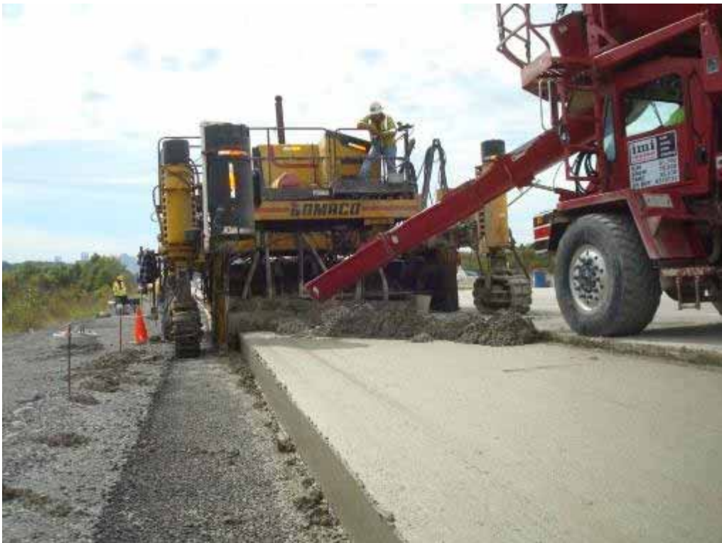
Photo E-26. Placement of top lift concrete by ready-mix truck chute.
