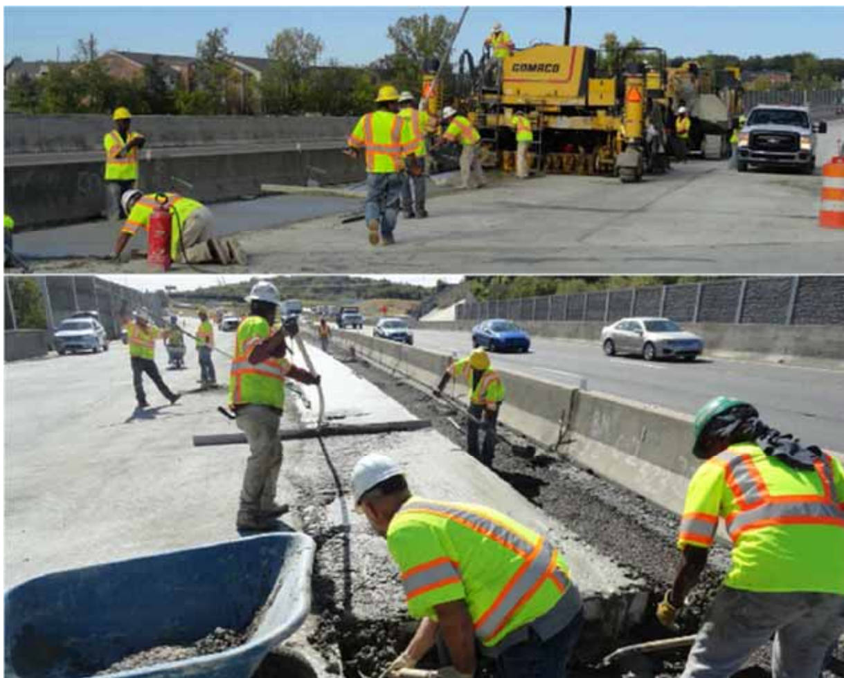
Figure 16: Construction of the shoulder using the conventional mixture
