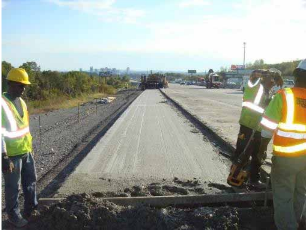
Photo E-35. Construction of Day 1 header (prior to top lift placement).
