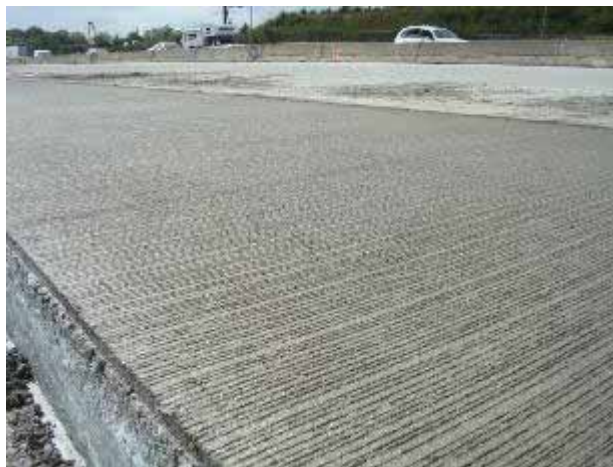
c. Completed transverse tining
