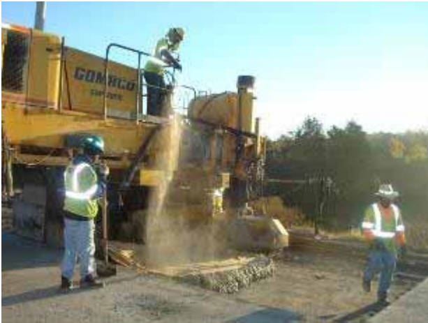
a. Watering burlap on bottom lift.
