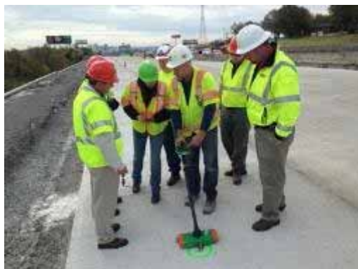
Figure 50: MCL staff measuring Pavement Thickness using the MIT
