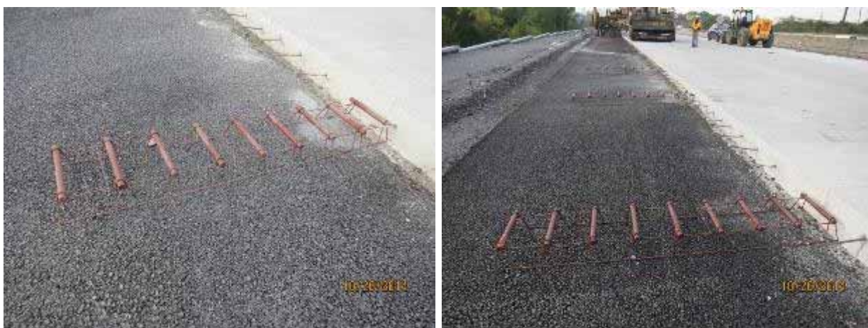
Figure 6. Dowel bar and tie bar configuration.
