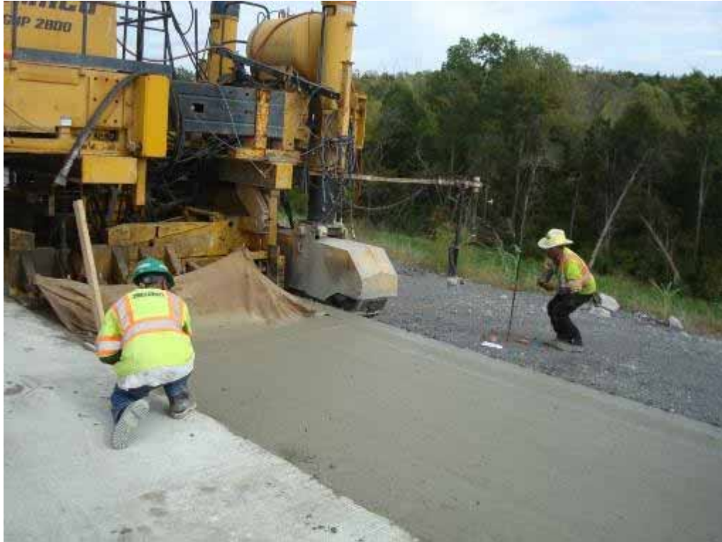
Photo E-19. Workers checking bottom lift elevation and profile using stringline.
