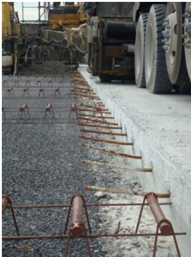
Photo E-14. Dowels and tie bars ahead of first paver.
