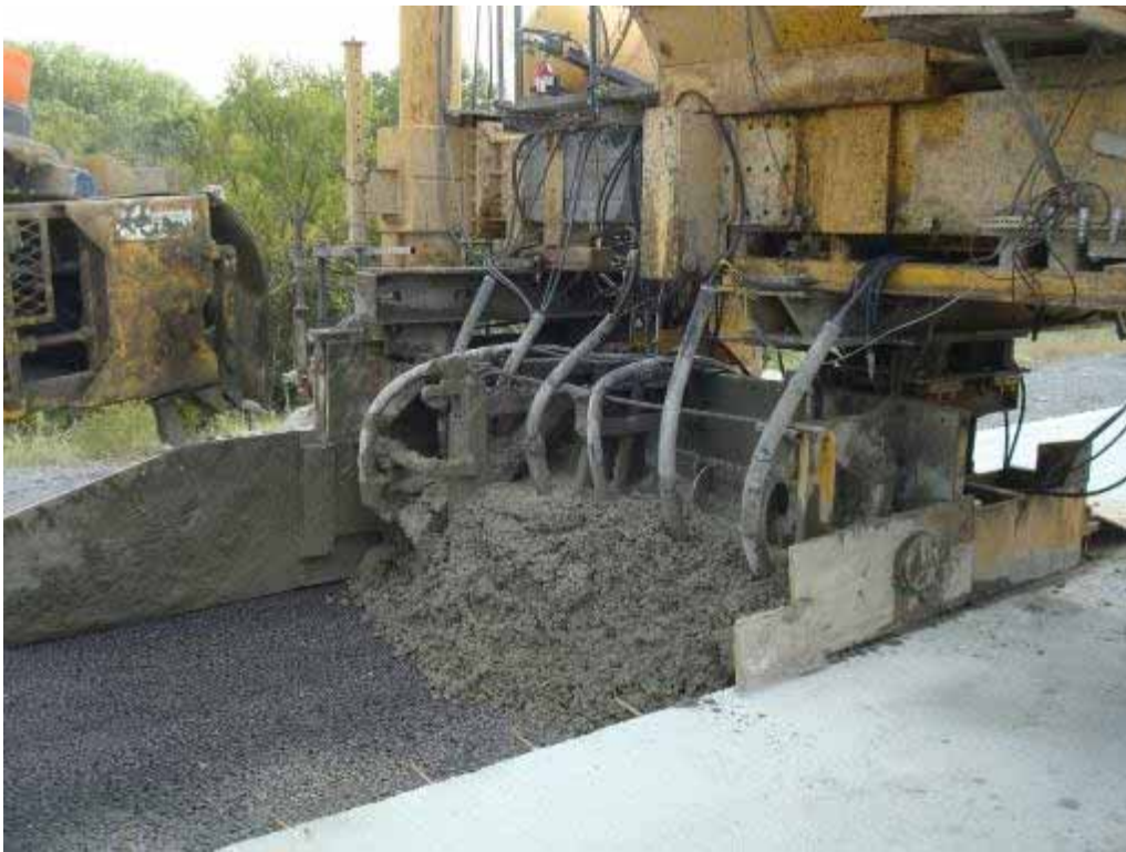
Photo E-16. Paving operation – bottom lift, front view.
