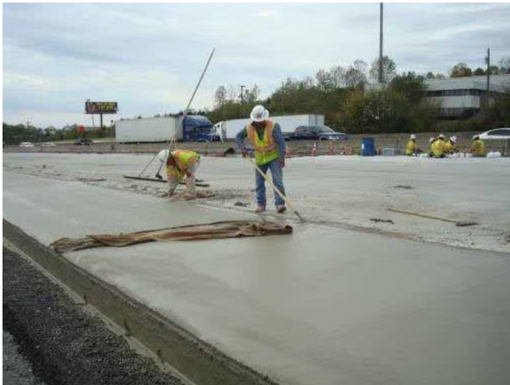
Photo E-48. Workers using edging tools to create lane-shoulder joint.
