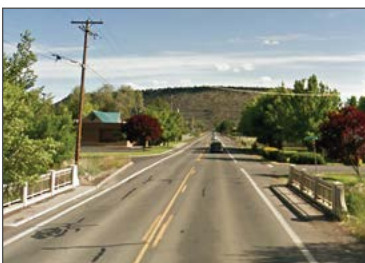
Ochoco Bridge project in Prineville, OR used in R09 demonstration workshop.
