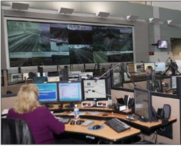
Staff in the McConnell Public Safety Transportation Operations Center monitor roadways in northern Virginia. (Photo courtesy McConnell Public Safety Transportation Operations Center.)
