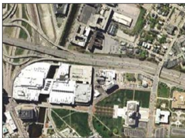
The I-95 Northbound Viaduct in Providence, RI.
