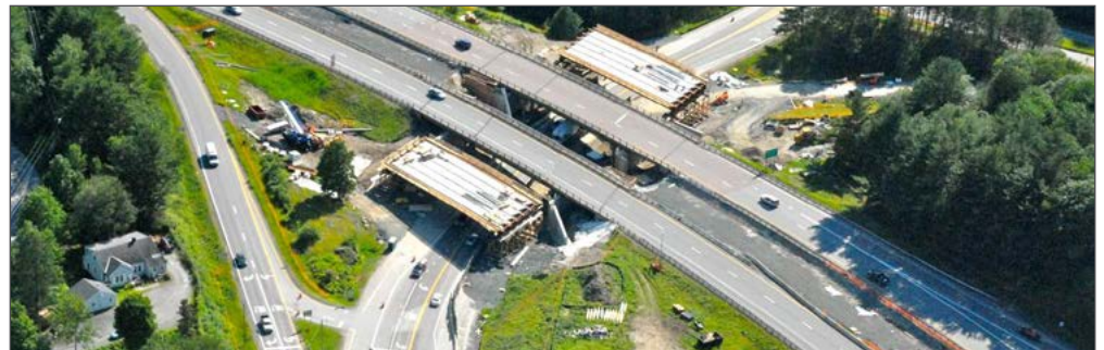
Hartford lateral slide bridge on I-91. (Photo courtesy VTrans.)
