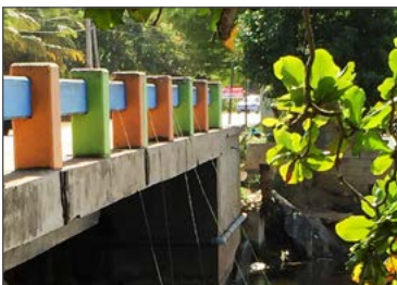
Bridge 702 on Puerto Rico Route 681 before Arecibo, Puerto Rico.
