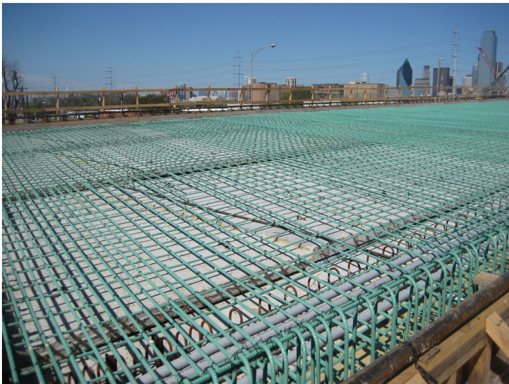
Figure 2. Photo. Typical PDDP installation prior to cast-in-place topping.
