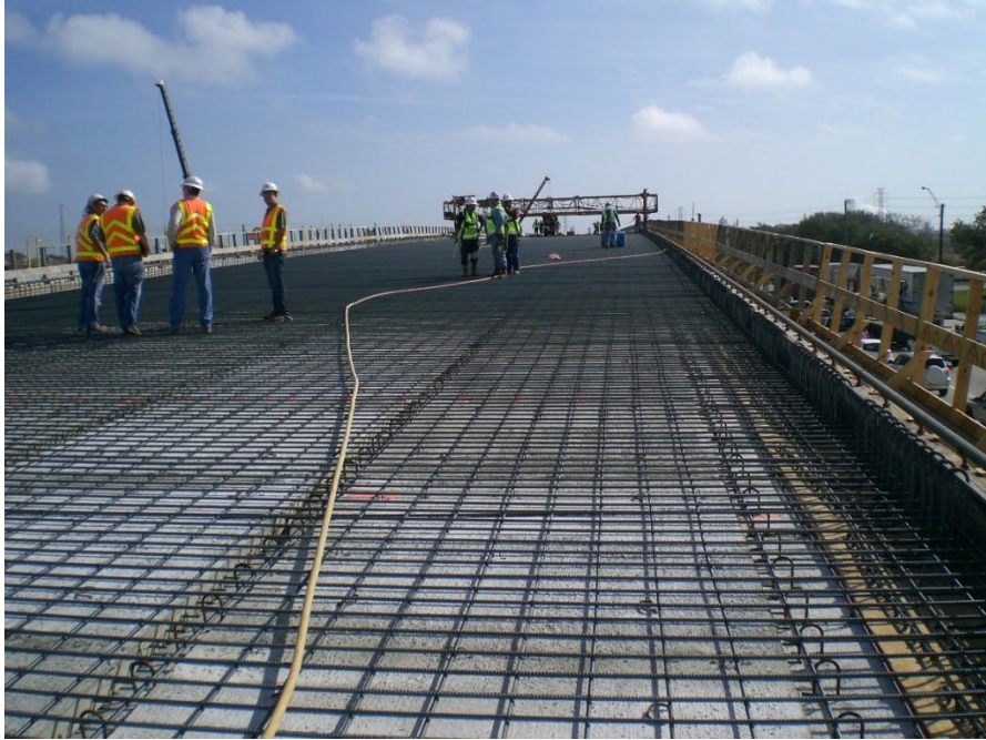
Figure 38.Photo. Deck ready for CIP concrete.
