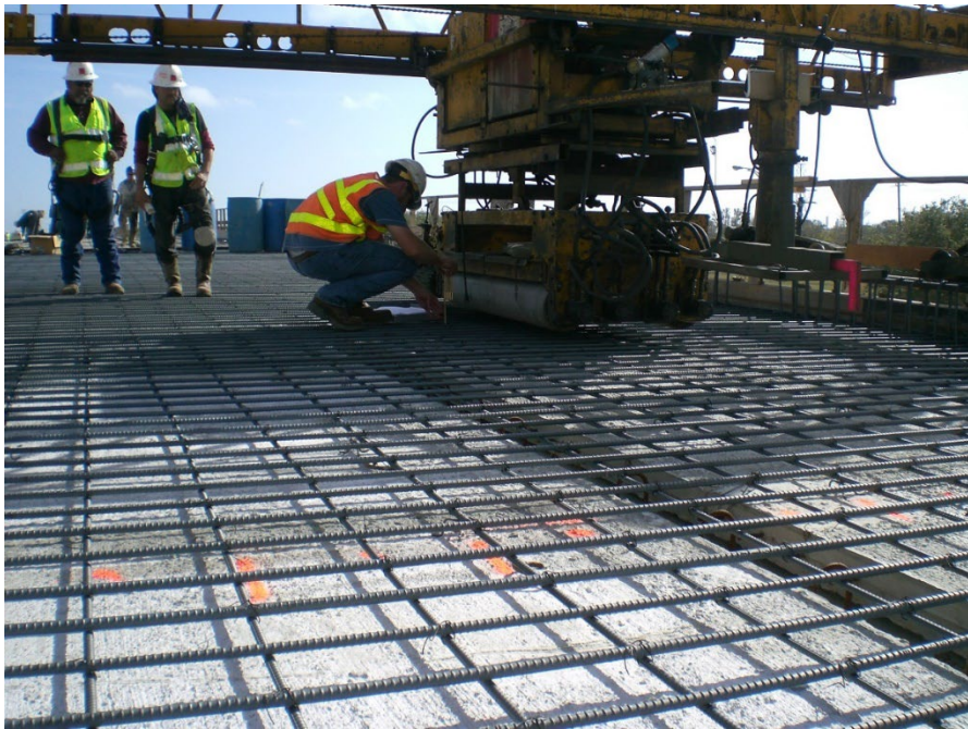
Figure 39.Photo.Screed used to strike off CIP concrete.
