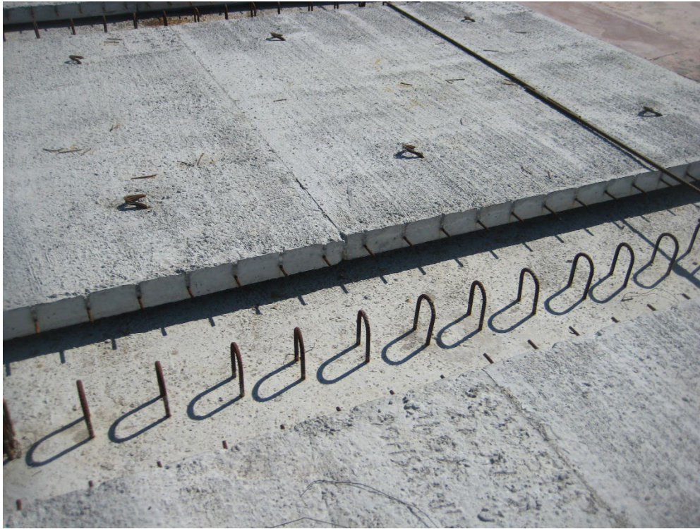
Figure 27. Photo. Roughened surface of PDDPs and top of girder.
