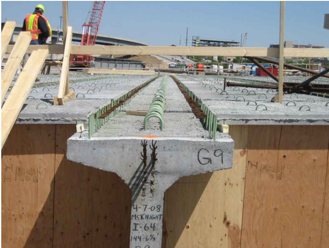
Figure 24. Photo. Semi-flexible temporary supports.
