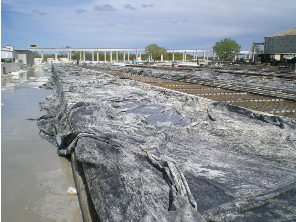
Figure 33.Photo. Curing of PDDPs using plastic sheeting.
