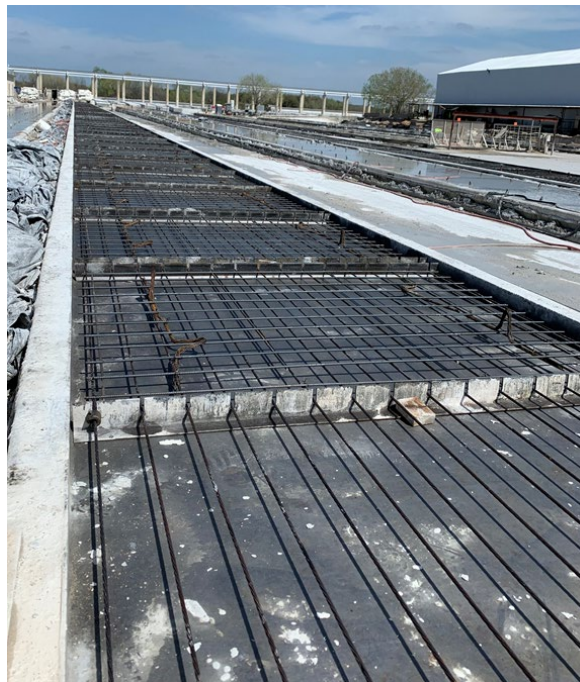
Figure 30. Photo. Forming of PDDPs
