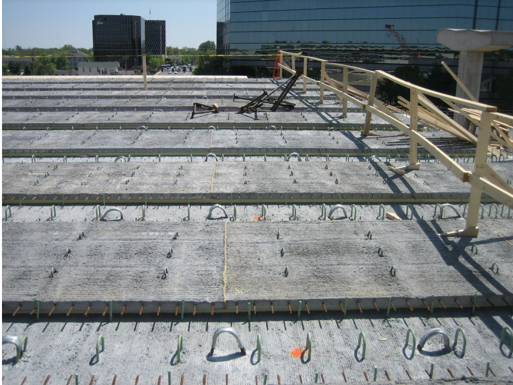
Figure 3. Photo. PDDP's in place providing a safe work zone.
