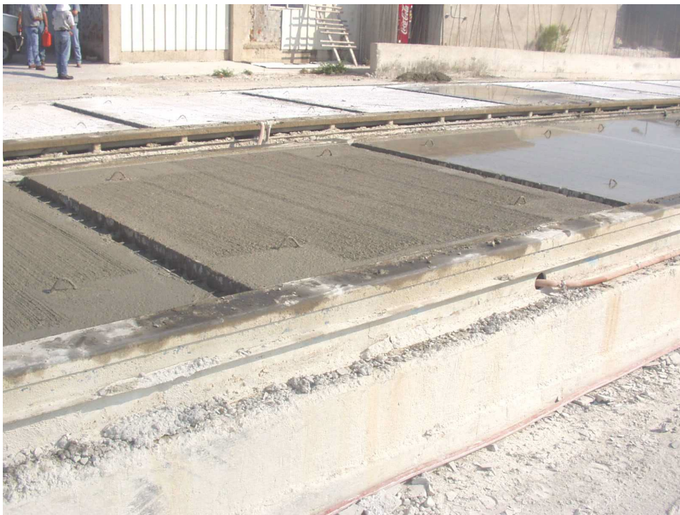
Figure 34.Photo.PDDPs after removal of plastic sheeting.
