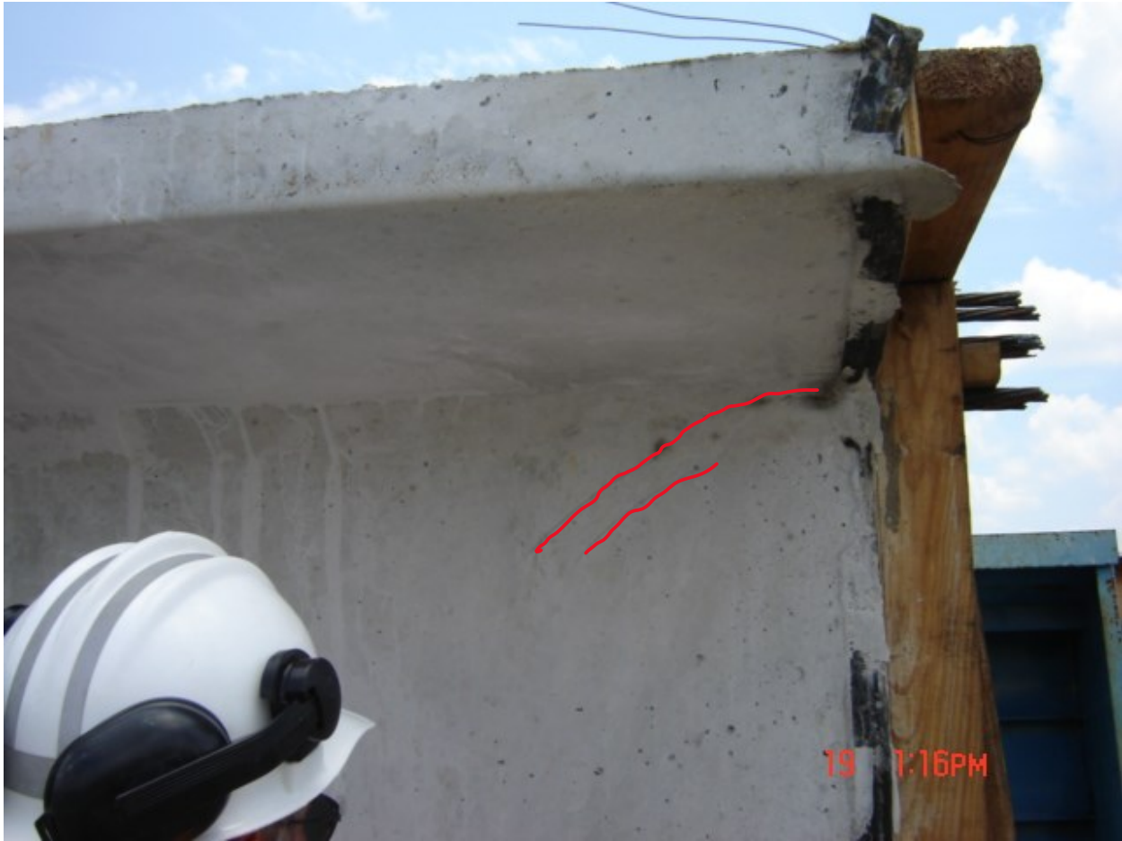
Figure 14. Example of cracking related to prestress transfer.
