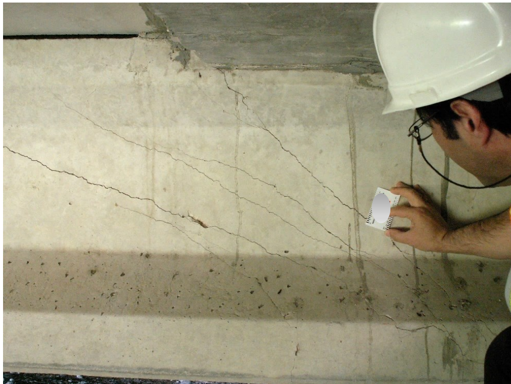
Figure 11. Shear cracks in a prestressed I-girder).
