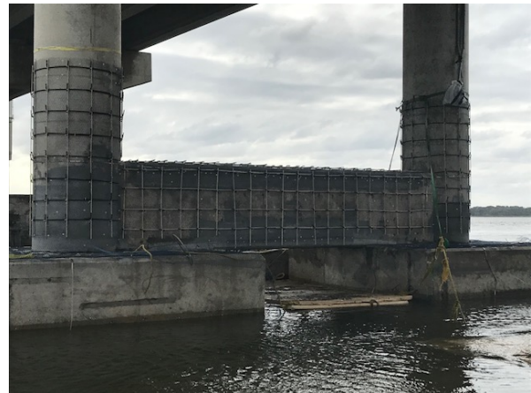
Figure 16. Photo. Crescent Beach concrete repairs completed, titanium mesh and reinforcement in-place, prior to forming and concrete placement.
