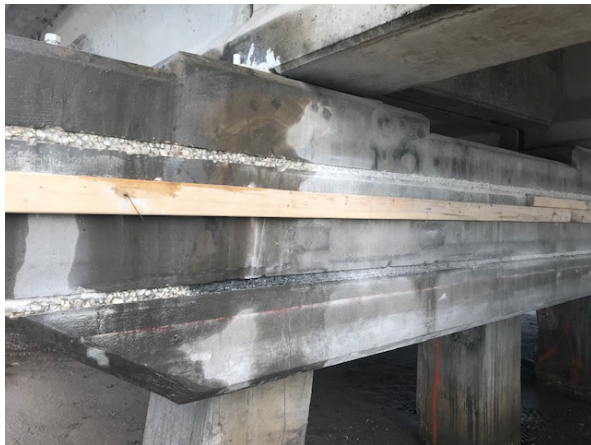
Figure 15. Photo. Crescent Beach excavation for titanium ribbon installation.
