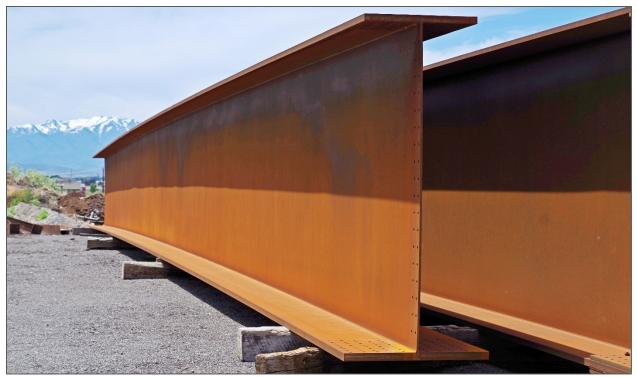
Figure 49: Photo. Fabricated steel plate girders for the I-80 bridges.
