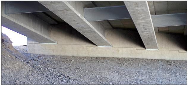
Figure 55: Photo. Constructed abutment on SR 36 bridge.
