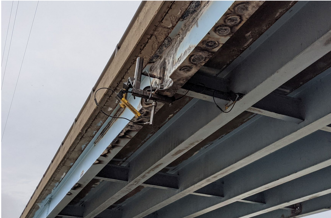
Figure 49. Photo. Jacks in place on an Indiana Bridge
