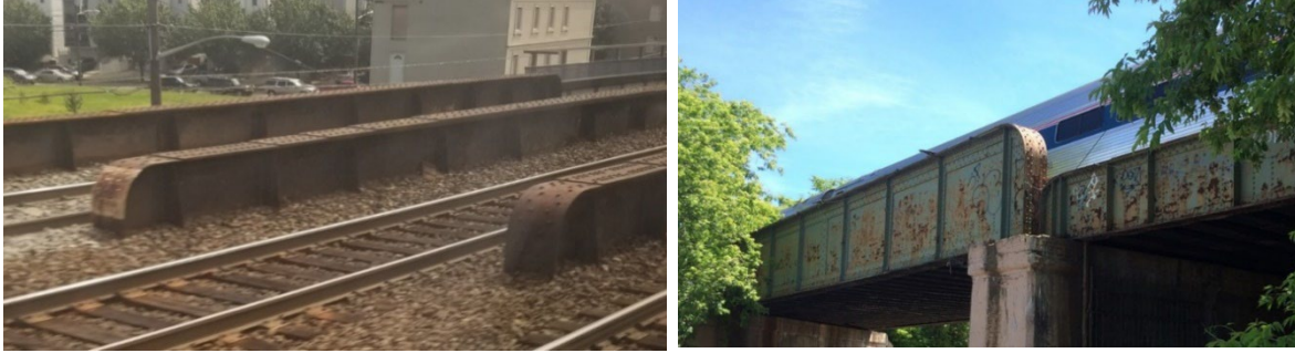
Figure 124. Photos. Railroad bridge girders with turned-down flanges.
