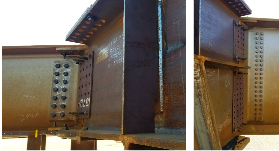
Figure 128. Photos. Cold-bent connection plates.
