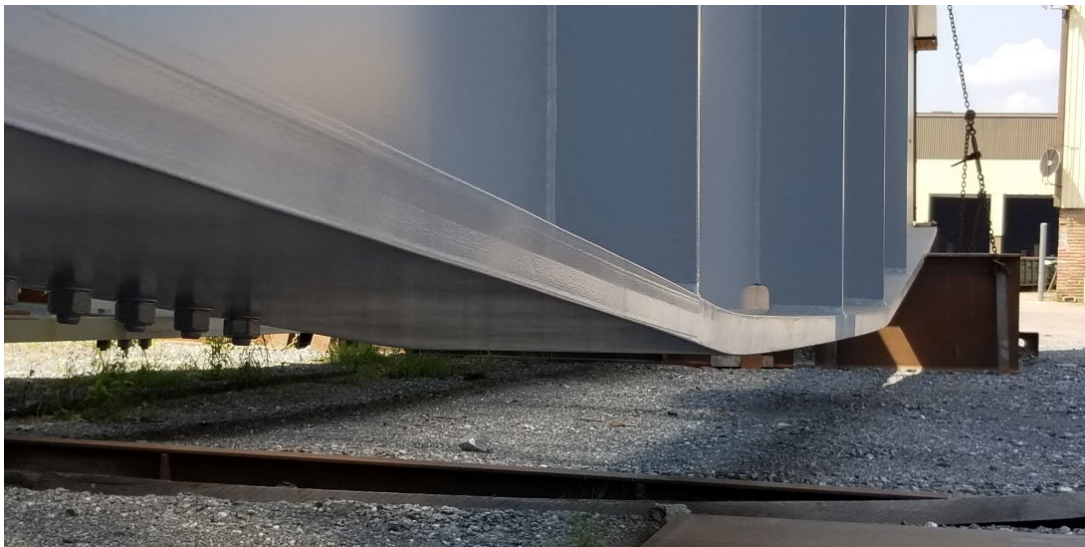
Figure 122. Photo. Cold-bent flange corner on haunch girder.
