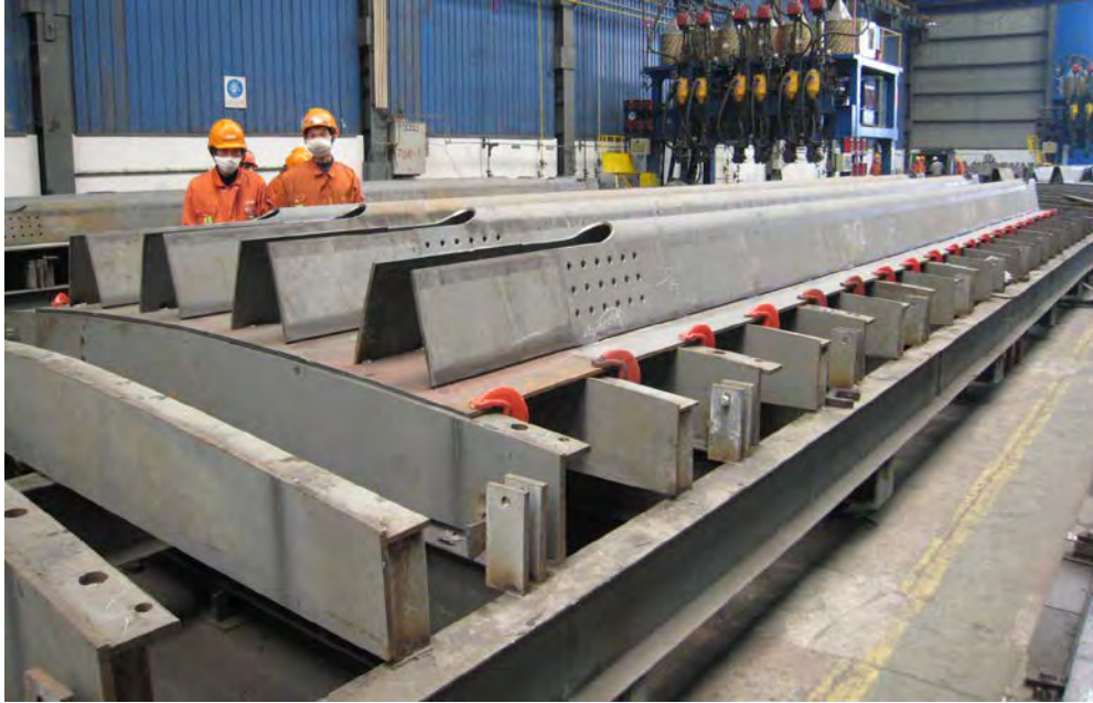
Figure 7-3 Pre-bending by Clamping the OSD to a Curved Assembly Bed is used to Offset Deck Panel Distortion due to Welding
