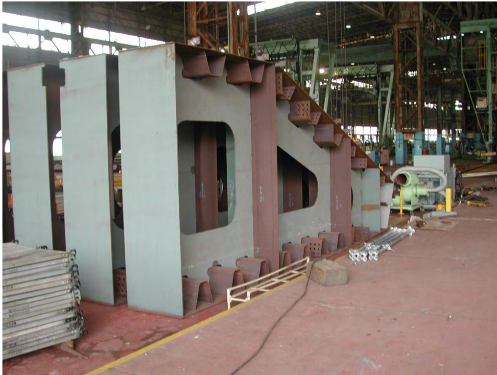
Figure 7-4 Fit-up Fixtures such as the One Shown for a Box Girder are Used To Ensure Alignment without Assembly
