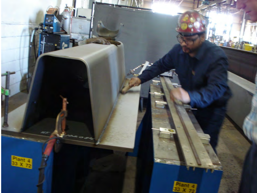
Figure 7-6 The Fabricator will Develop a Procedure for Rib-to-Deck Welding as the Worker in the Photo is Testing
