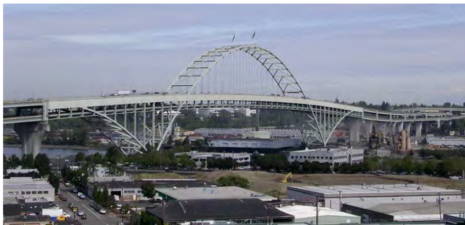
Figure 2-3 Photo of the Fremont Bridge over the Willamette River in Portland, OR. The Upper Deck is an Orthotropic Steel Deck for the Full Length of the Main Span Unit.
