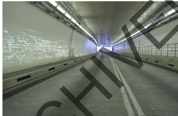
Figure 7-1: Tunnel with transverse ventilation showing ducts.
