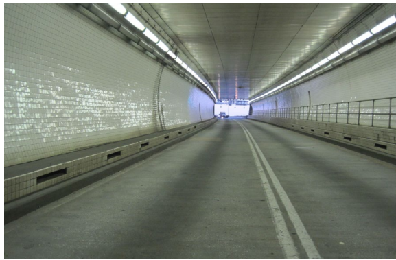
Figure 5-33: Tunnel with transverse ventilation showing ducts.
