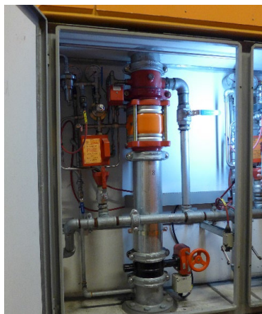
Figure 4-3: Deluge valve cabinet arrangement [15].
