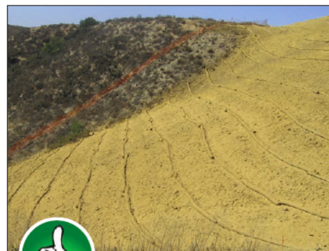
Fig. 1-1. Proper management of construction sites through the use of BMPs can dramatically reduce stormwater impacts. Source: RBF Consulting
