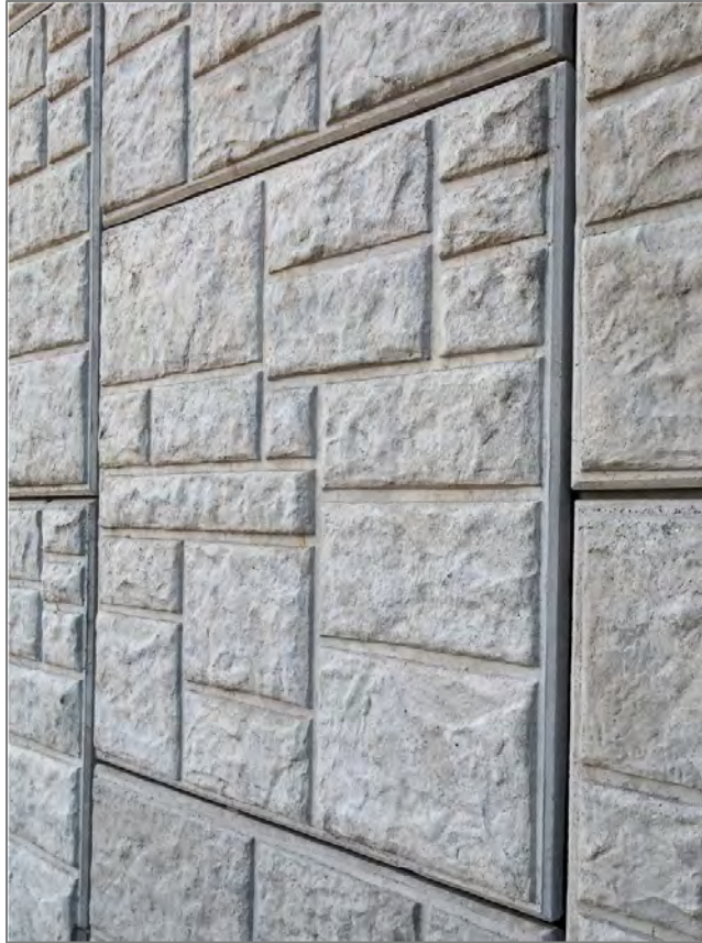
Figure 7: SCP facing (Courtesy RECo)
