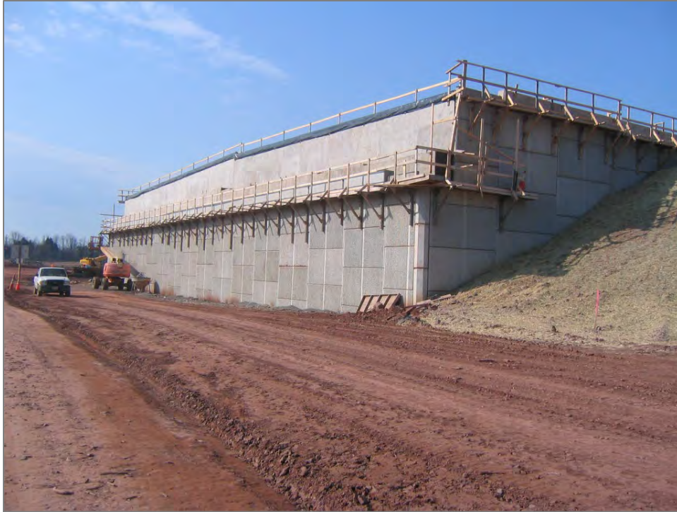
Figure 29: Construction of traffic barriers and copings
