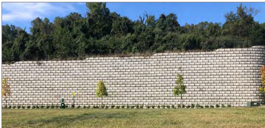
Figure 2: MSE wall for grade change
