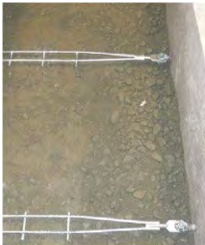
Figure 12: SCP and two-wire steel strip reinforcement connection
