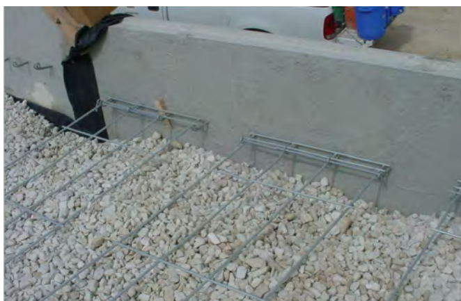
Figure 13: SCP and steel wire grid reinforcement connection
