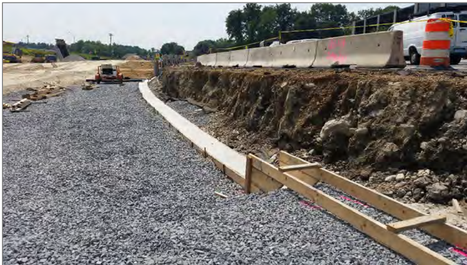
Figure 24: Placement of leveling pad
