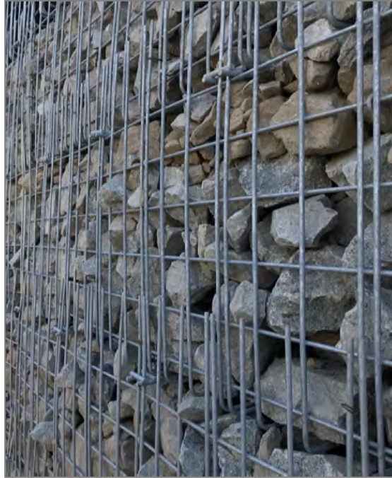
Figure 10: Flexible facing system (Courtesy AIL)
