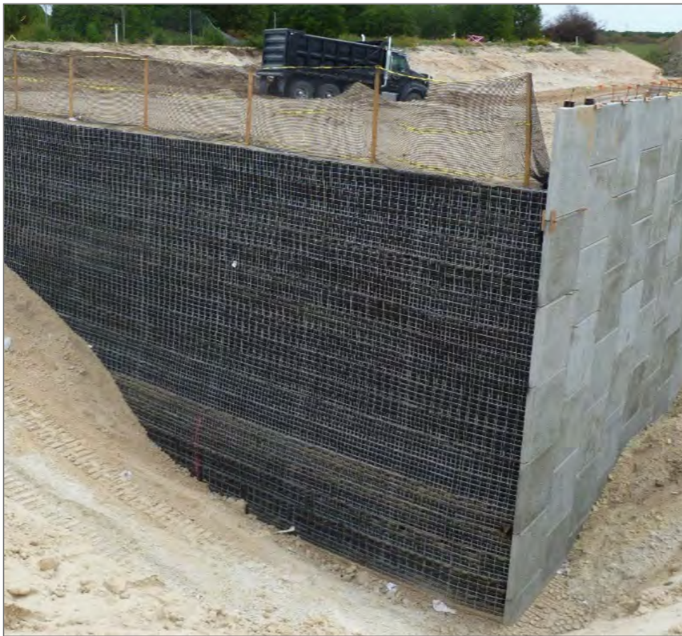
Figure 6: Temporary MSE wall for phased construction
