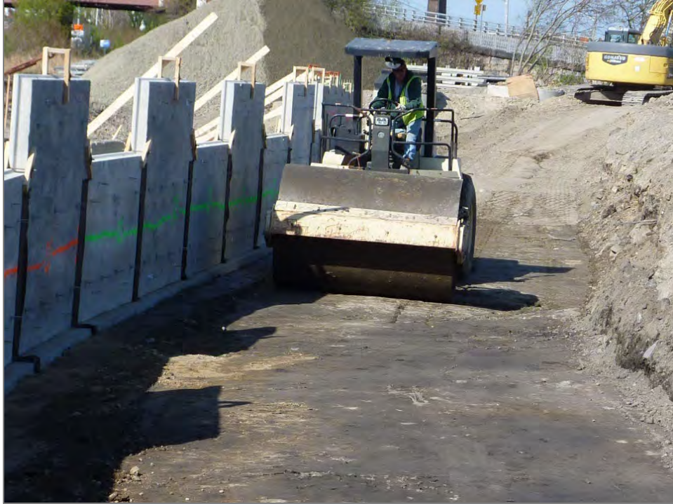
Figure 23: Preparation of subgrade
