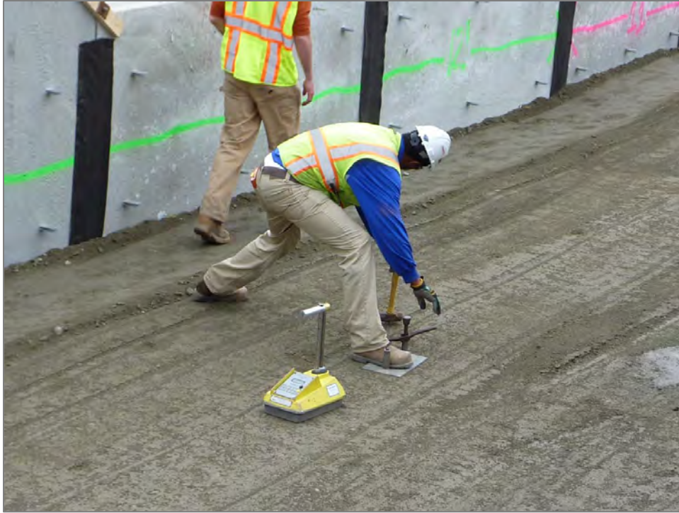
Figure 27: Checking fill density
