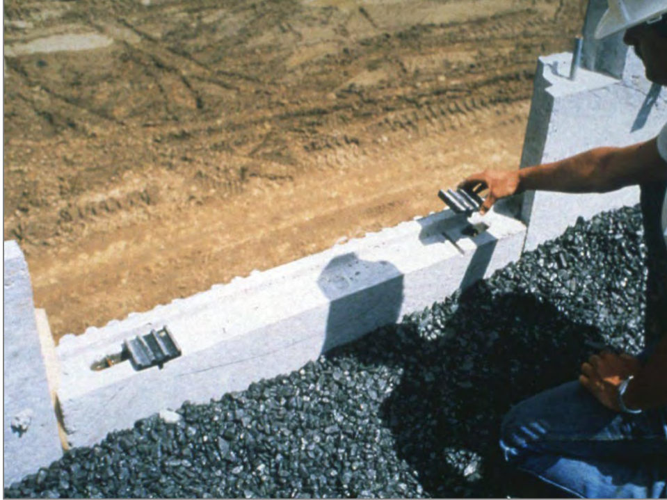
Figure 21: SCP bearing pads
