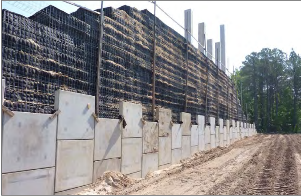
Figure 5: Two-stage MSE wall
