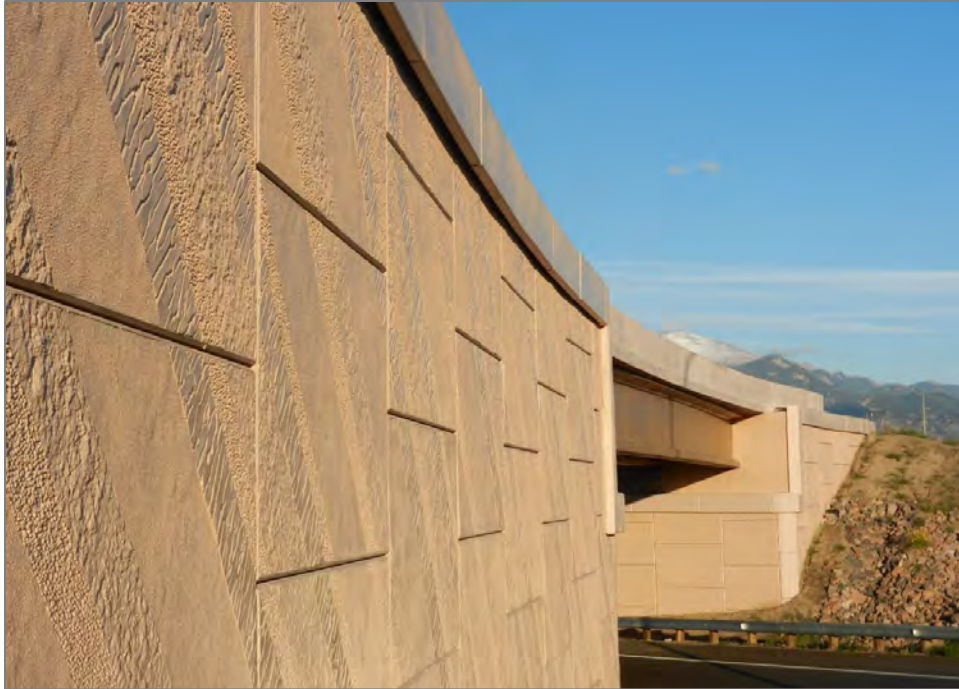
Figure 3: MSE wall for bridge abutment
