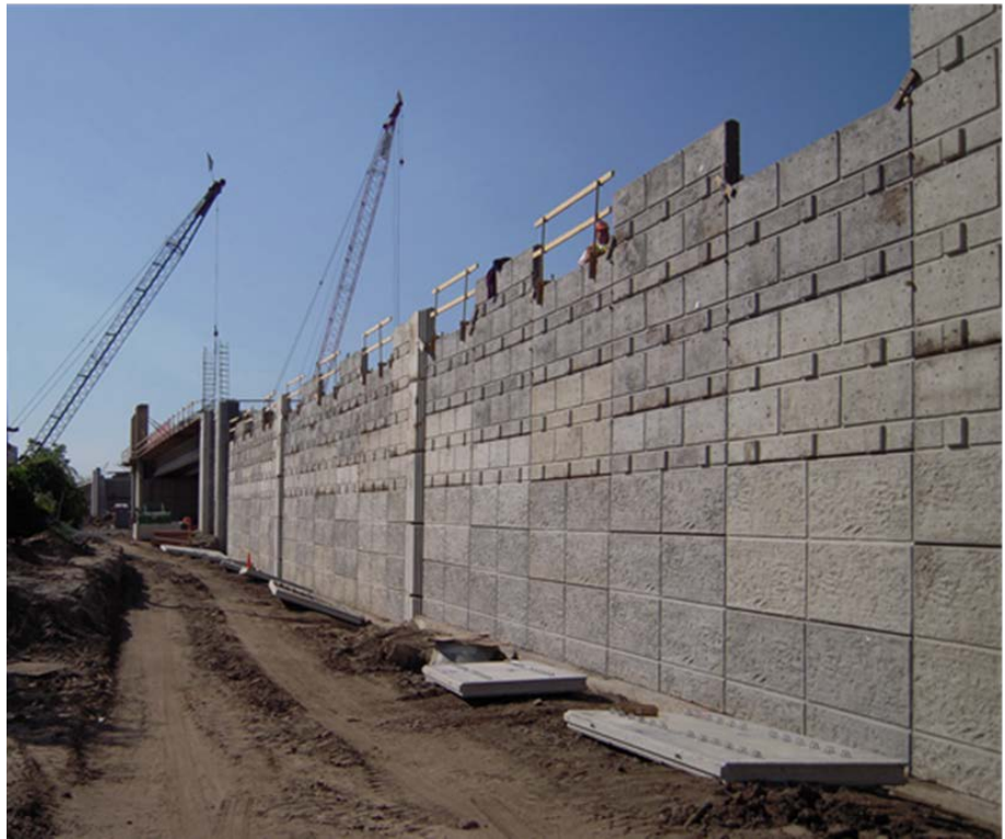
Figure 10-4. MSE wall construction on MnDOT Crosstown Project.
