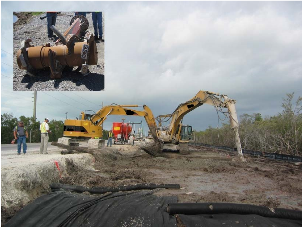
Figure 7-3. Mass mixing; inset shows close-up of a mass mixing tool.
