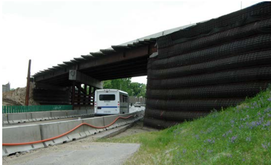
Figure 10-6. MSE walls to support temporary bridge abutment and roadway embankment.
