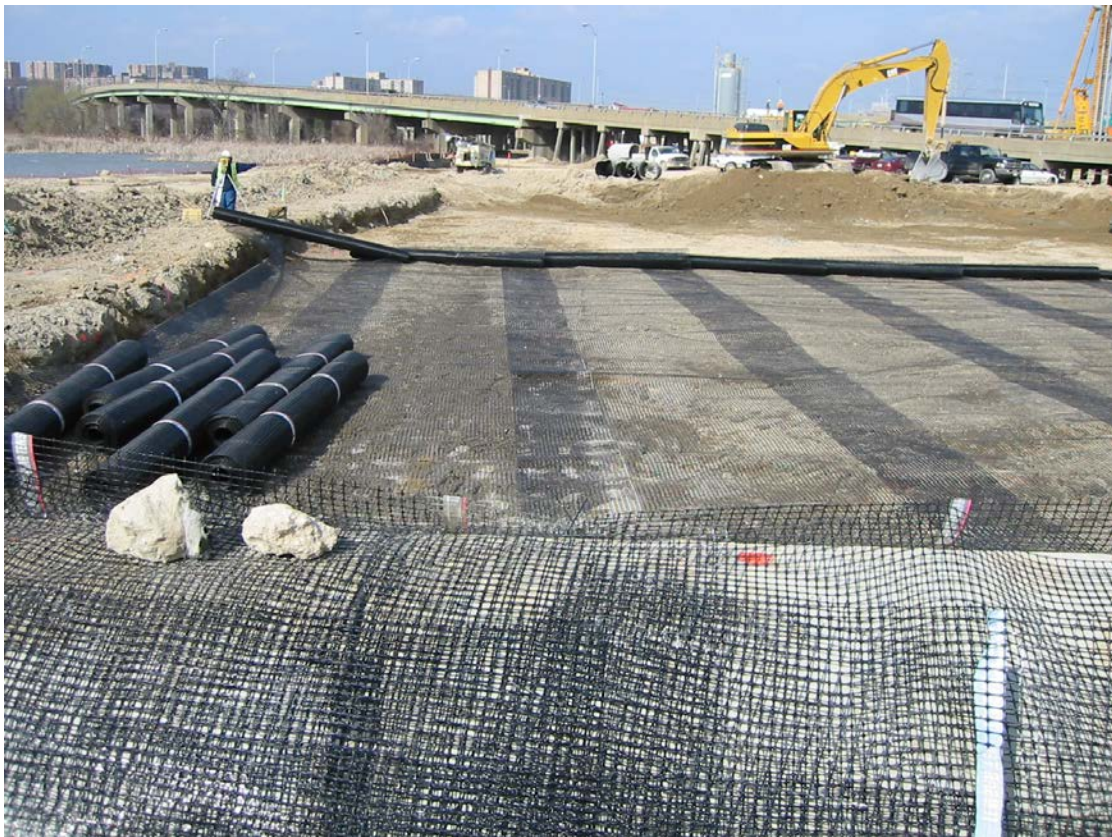
Figure 6-6. Load transfer platform reinforcement placement.
