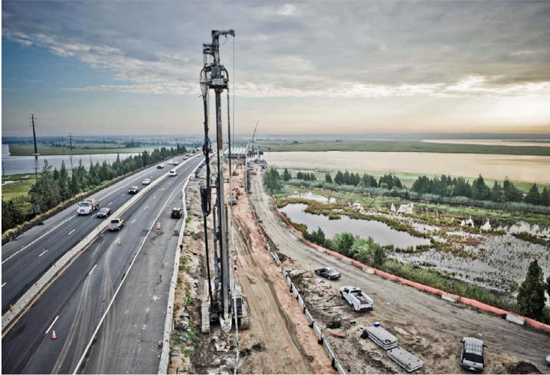
Figure 6-18. CMC installation Phase 2.
