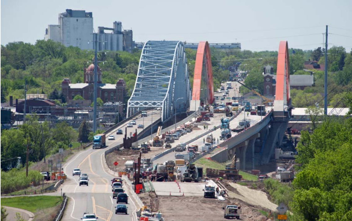
Figure 6-22. Completed north approach embankment and approach spans, US 61.
