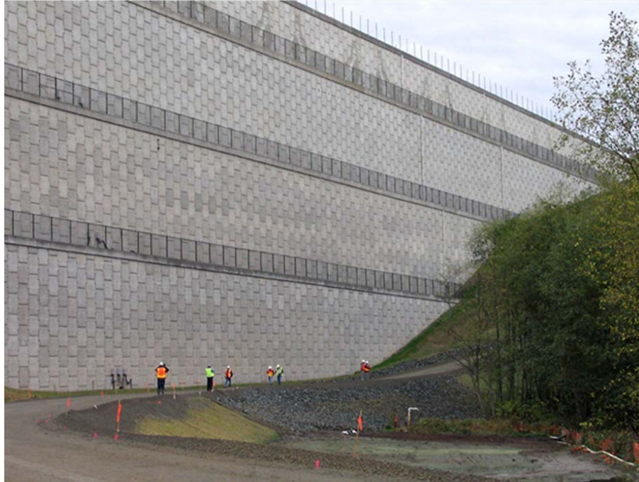
Figure 10-5. SeaTac Airport runway extension MSE wall.
