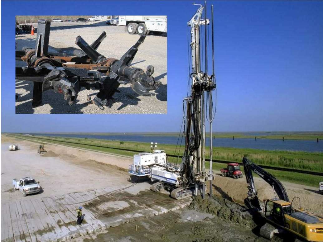
Figure 7-1. Deep mixing by the wet method; insert shows double-axis mixing tool.
