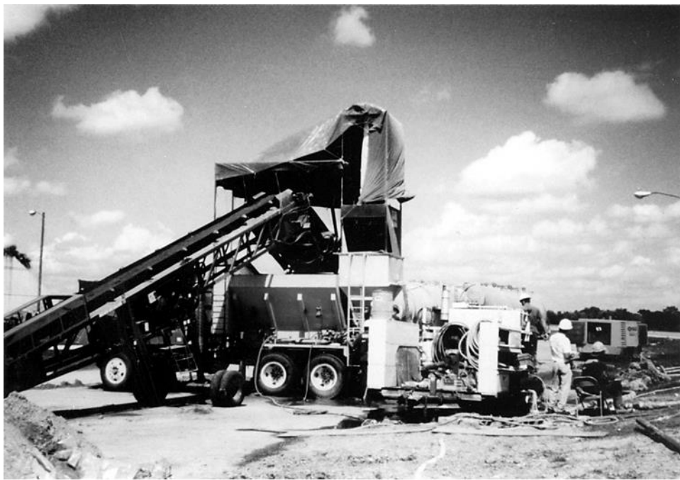
Figure 8-40. Larger on-site grout batching plant for compaction grouting.
