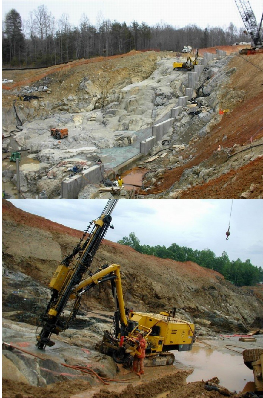
Figure 8-29. Grouting operations at Hunting Run Dam, Virginia.
