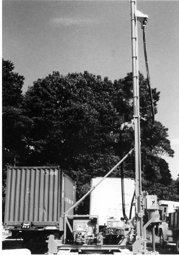
Figure 8-43. Jet grouting rig.
