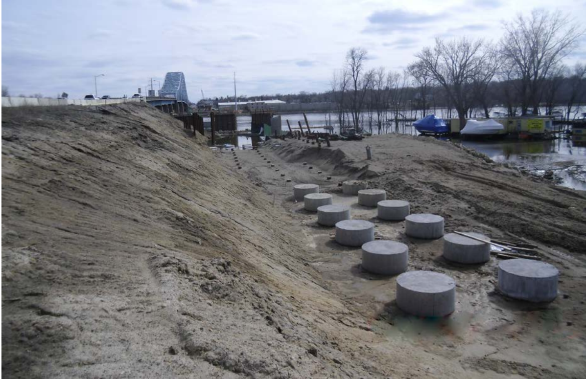
Figure 6-21. Pile columns and (near) pile caps installed, US 61.
