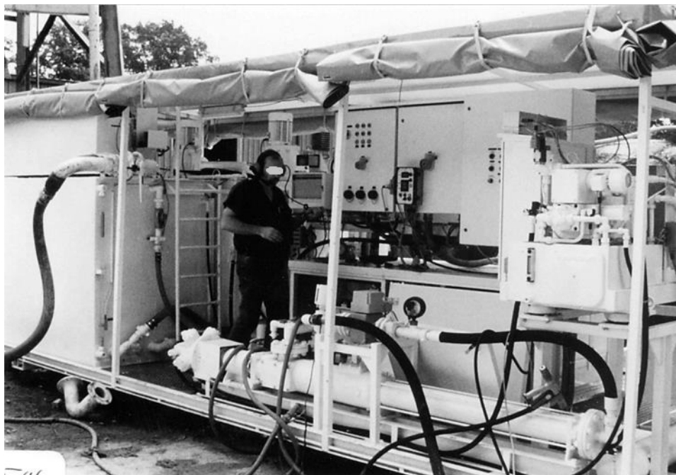
Figure 8-45. Pumping station for HMG grouting.
