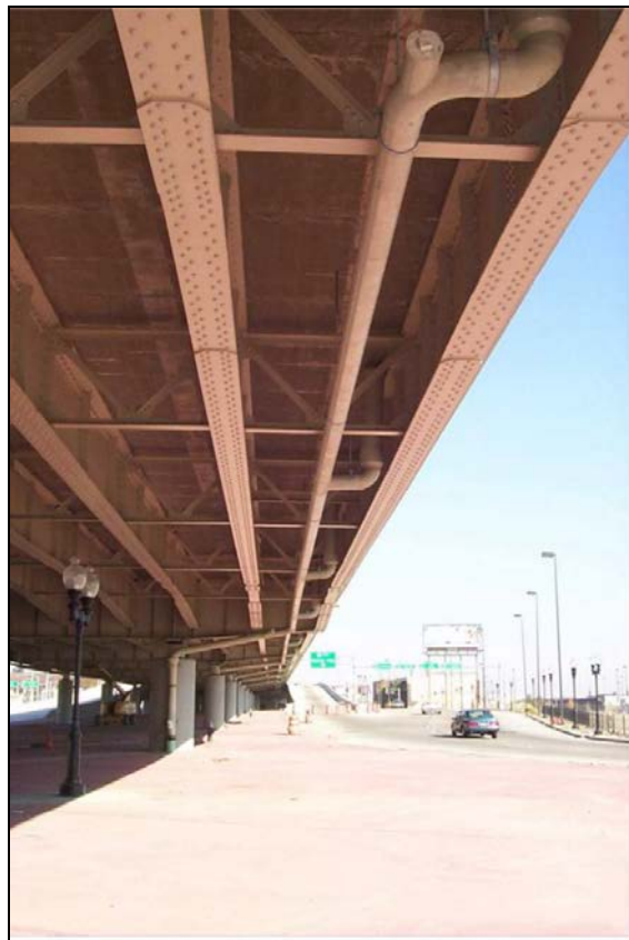
Figure 10.14. Installed underdeck bridge drainage system.
