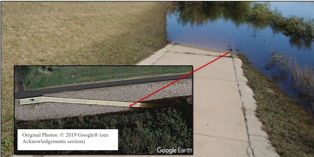
Figure 6.9. Site photo of high-water line and associated orthoimage.
