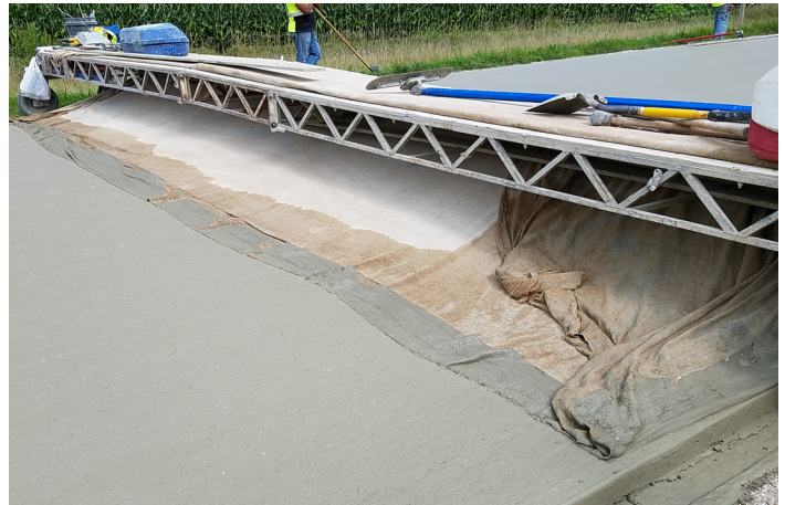
Fiber-reinforced concrete overlay with 4 lb/yd 3 of synthetic macrofiber and 4-in depth showing excellent finishability. Source: Iowa Concrete Paving Association (ICPA)
