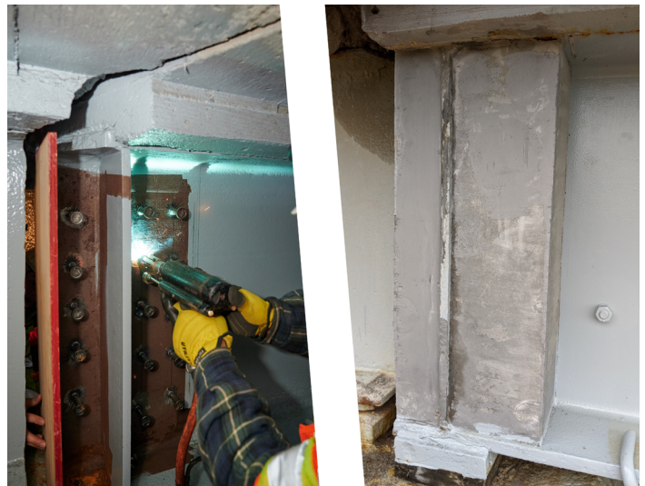
Repair of a deteriorated steel bridge beam end using UHPC.
