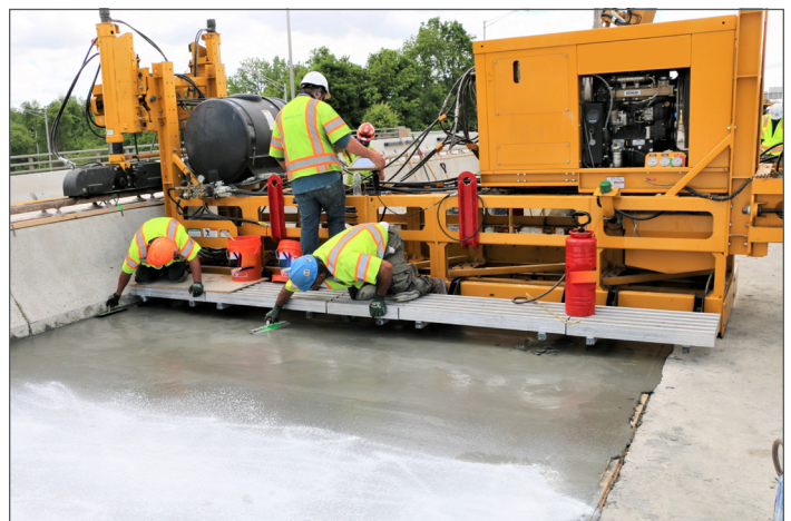
Installation of a UHPC overlay. Source: FHWA
