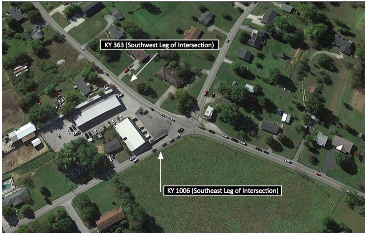
Figure 2 Aerial View of Four-Way Stop Intersection at KY 363 and KY 1006 Before Construction
