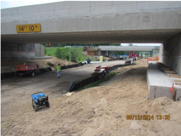
Figure 4 - Extended footing toe for overturning resistance
