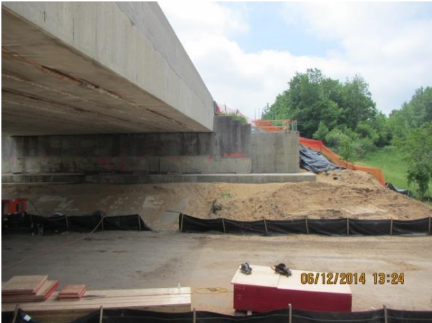
Figure 3 - Elevation view of the abutment extension
