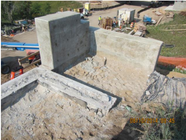
Figure 2 - Extension of abutment with new wing wall
