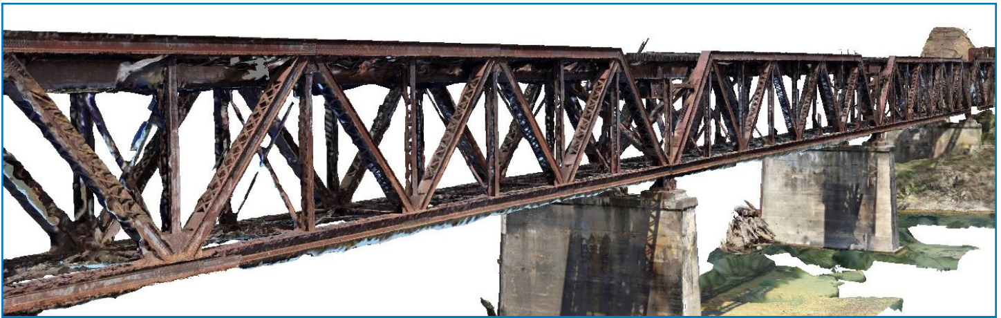
Example of a 3D model of a bridge produced using photogrammetry data from a UAS.
