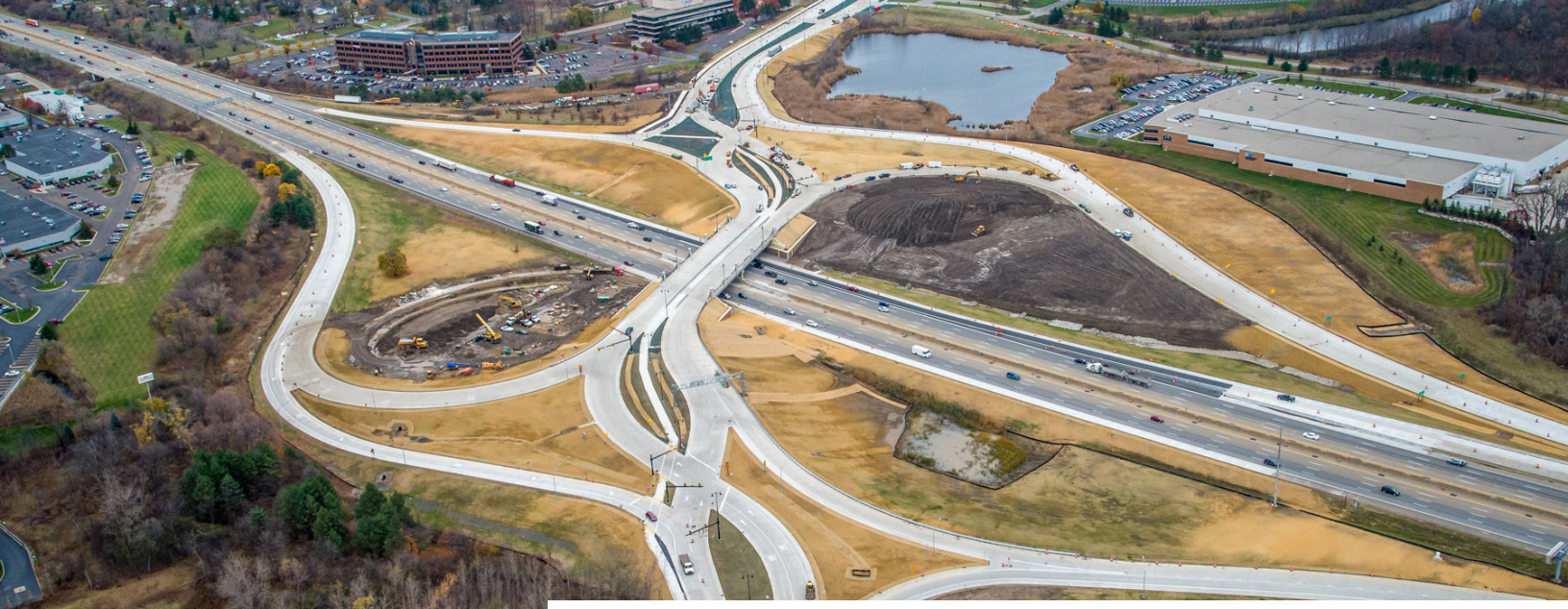
An unusual crossing angle saved money on Michigan's first diverging diamond interchange.
