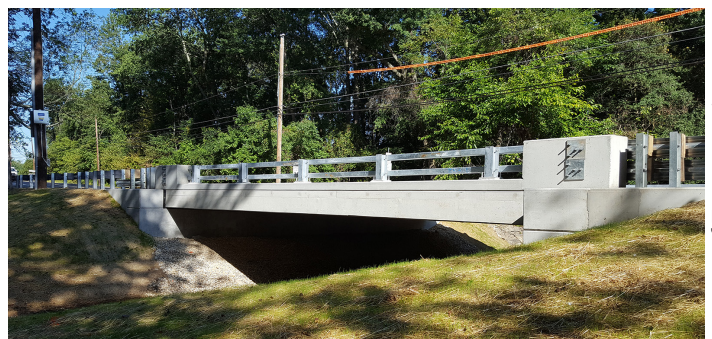
The Delaware Department of Transportation combined precast elements with UHPC connections and a UHPC overlay on an Accelerated Innovation Deployment Demonstration project.
