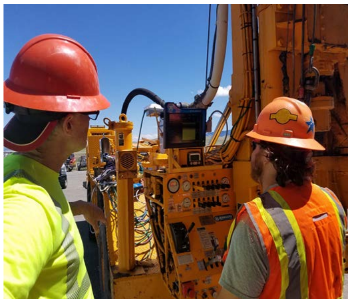
Credit: Montana Department of Transportation
