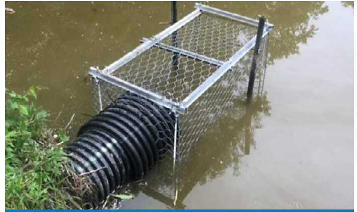
The beaver pipe cage keeps the animals from packing culverts with sticks and mud.
